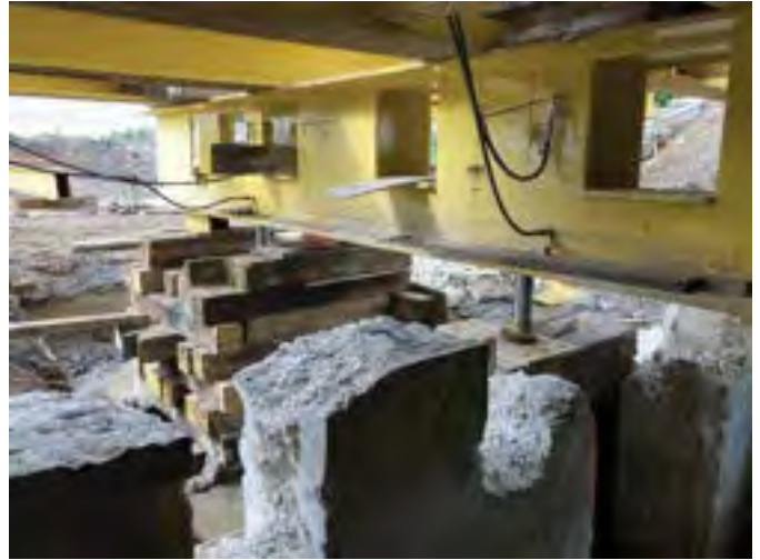
Integrated synchronized hydraulic jacks in main beams
