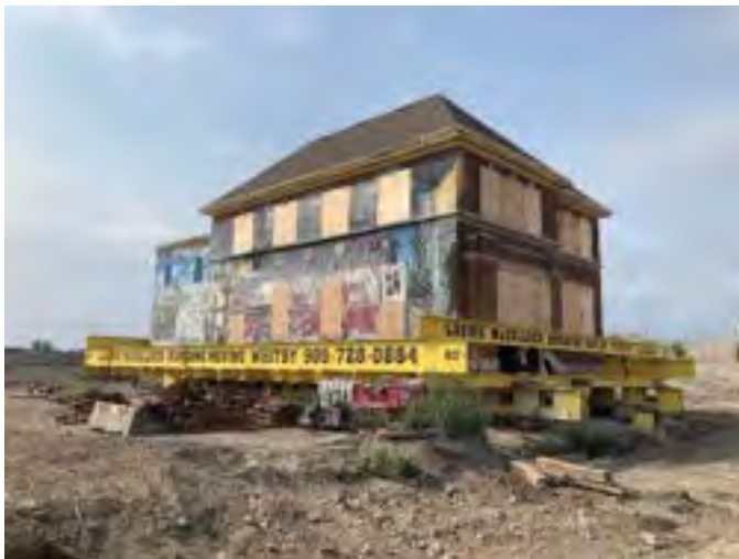
Relocated and positioned above new footings
