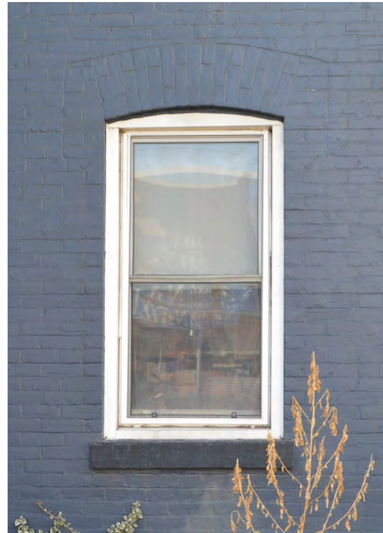
Above: Typical window opening with new aluminum window frame retrofitted inside what is believed to be the original wood frame, covered in metal cladding.
