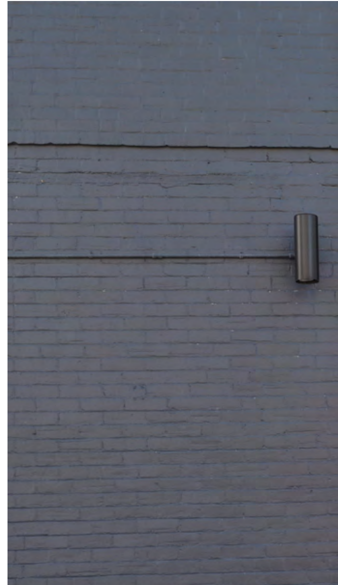
Above: Close-up of masonry concealed beneath blue paint.
