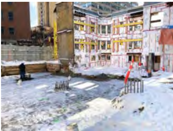
Retained Charles St façades and prep for depressed slab
