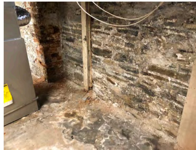
Below: Exposed stone showing poor condition of mortar joints.
