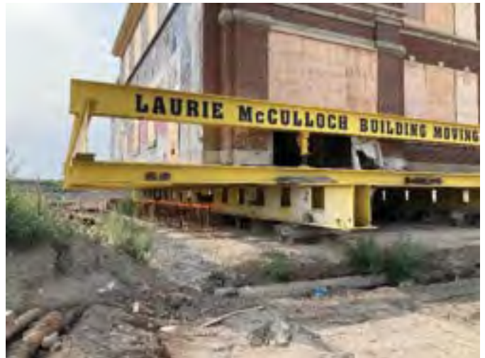
Supported on timber cribs prior to construction of Cast-in-place and CMU foundation walls
