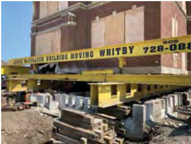
Separated from foundation, move in progress
