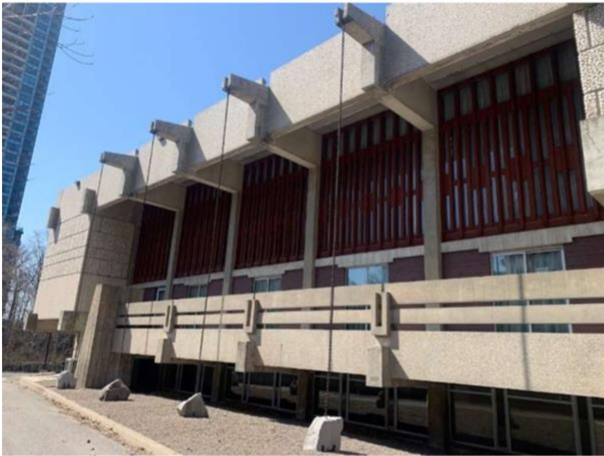
East elevation showing concrete roof troughs with suspended rain chains (kusari-doi) (Heritage Planning)
