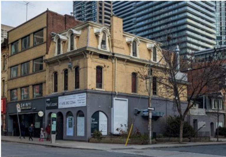
639 Yonge St. south and west elevations
