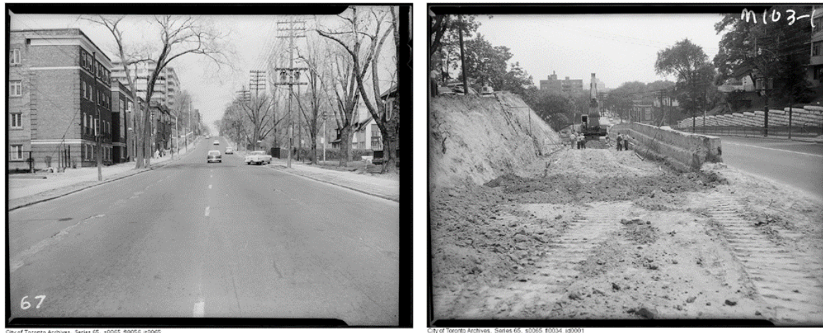
Figure 2: Avenue Road in early 20th century (left) and during the road widening project, 1959-60 (right), City of Toronto Archives
