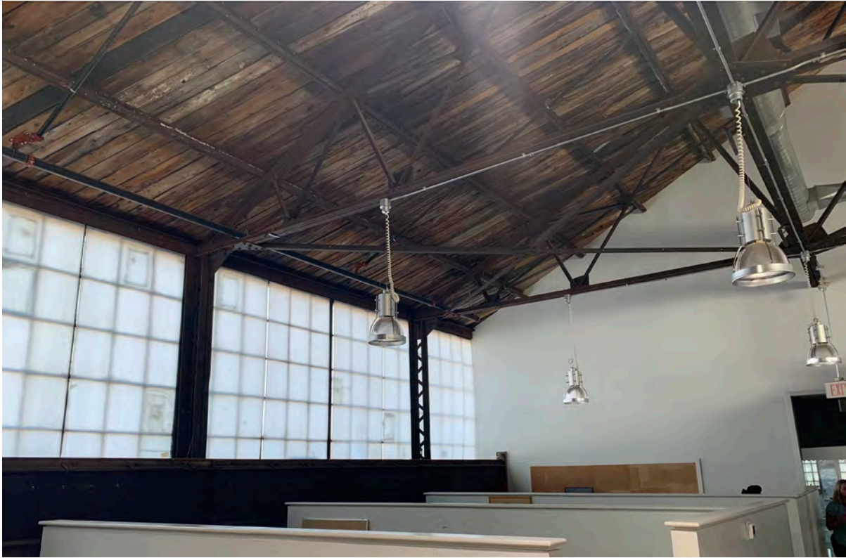
Figure 23. Interior looking northwest showing the clerestory windows and open span roof of the southern portion of the building (ERA, 2023).
