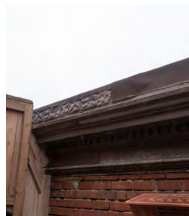
31. Units wrapped in bituminous membrane (Source: ERA).
