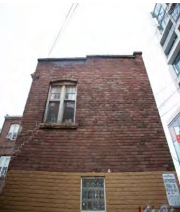
51. Concrete parapet cap is in poor condition (Source: ERA).
