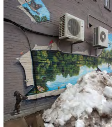
29. Painted plywood panels and erosion (Source: ERA).
