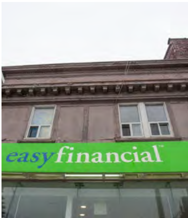
47. Infill panels within wood framing (Source: ERA).
