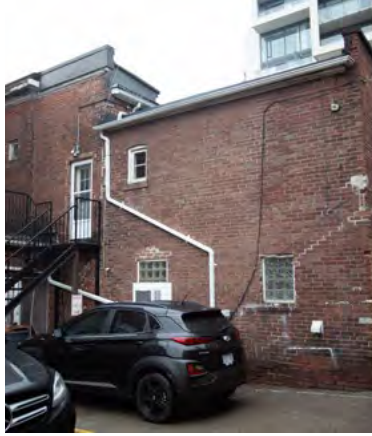
45. Rear parapets with warped cap to the east (Source: ERA).
