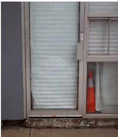
50. Deteriorating concrete at entrance (Source: ERA).
