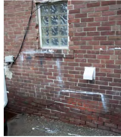
34. Large crack near grade (Source: ERA).
