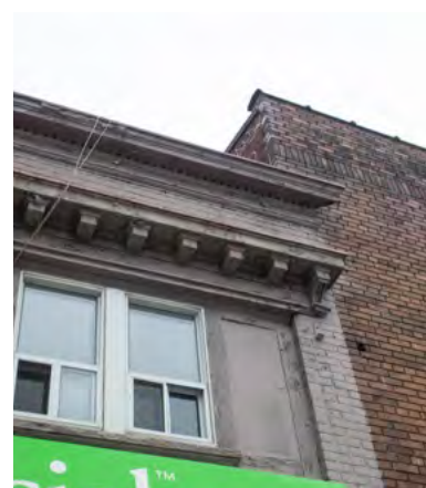
43. Painted tin cornice and modillions, west elevation (Source: ERA).
