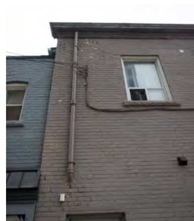
28. Large crack and plastic repairs on 2111 Yonge street (Source: ERA).
