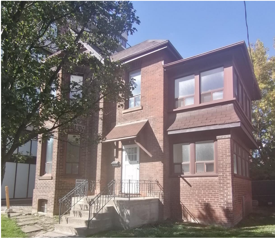
View of south and east elevations at 26 Millwood Road showing c.1926 2-storey enclosed porch (Heritage Planning, October 2024).
