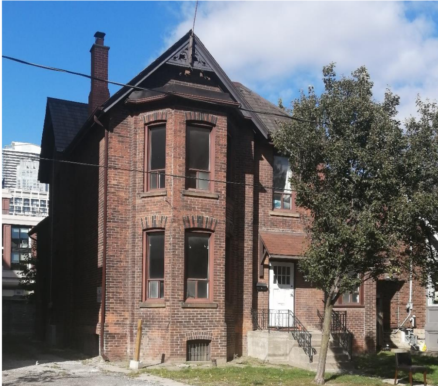
View of south and west elevations at 26 Millwood Road showing 2-storey 3-sided bay, brick voussoirs, stone sills and decorative gable pediments (Heritage Planning, October 2024).
