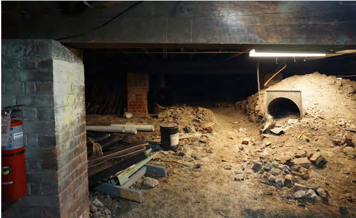
Sanctuary basement crawl space, showing unfinished floor, mechanical ducts and brick piers (ERA, 2022)
