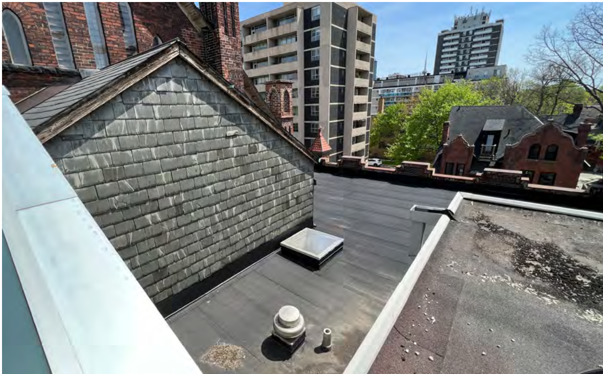
View from the 1889 Chapel/1913 Sunday School roof showing the condition of the sheet roofing used on the 1889 Chapel/1913 Sunday School and Link addition (ERA, 2022)
