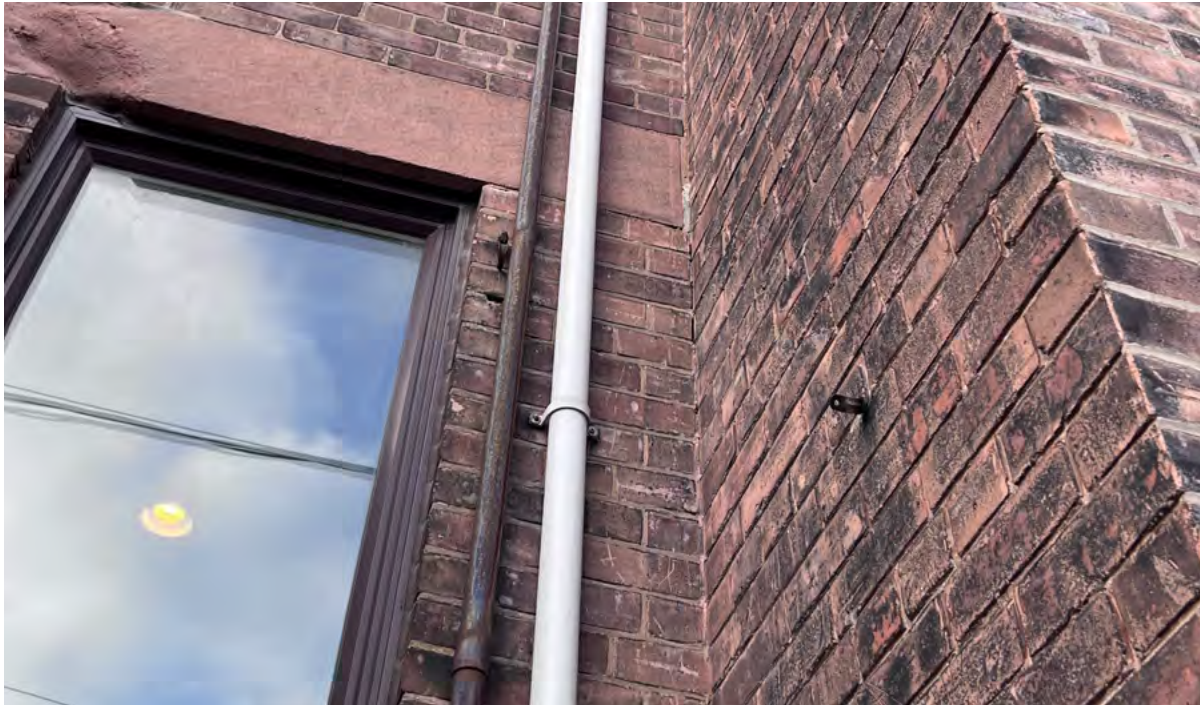
Link addition south elevation, featuring an entire replacement and infill of original windows , and replacement stone sills and headers that have spalled as shown (ERA, 2022)
