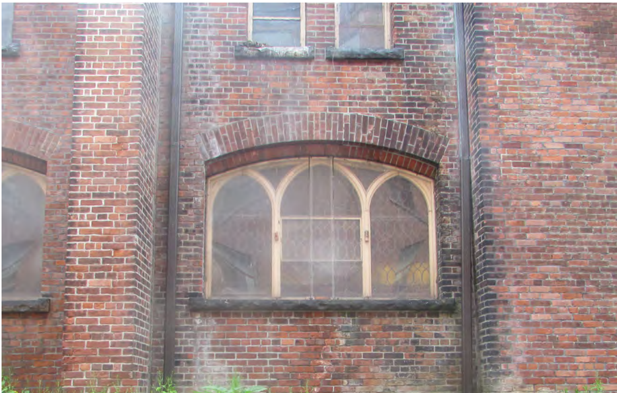
Sanctuary building north elevation, example of soiling at window openings and sills (ERA, 2022)
