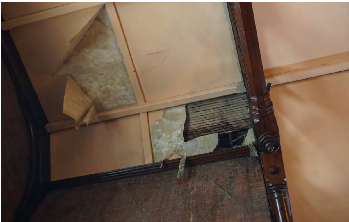
Sanctuary northeast interior corner, ceiling deterioration and efflorescence staining on the wall (ERA, 2022)
