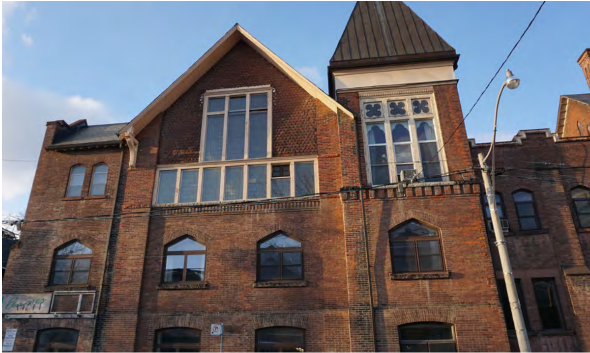
1889 Chapel/1913 Sunday School south elevation, showing replacement windows at ground and second floor and feature windows at the third floor (ERA, 2022)
