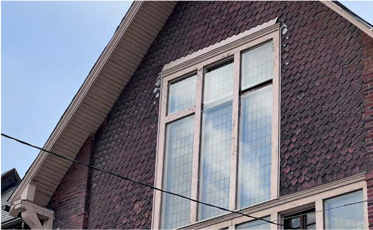
1889 Chapel/1913 Sunday School south elevation, terracotta tile with missing and wood replacement unit (ERA, 2022)
