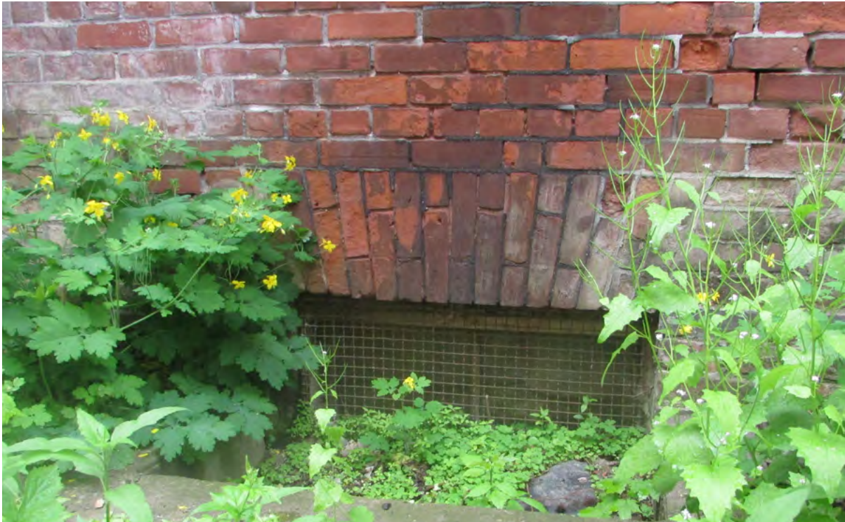
Sanctuary building north elevation, organic staining at basement level window well (ERA, 2022)
