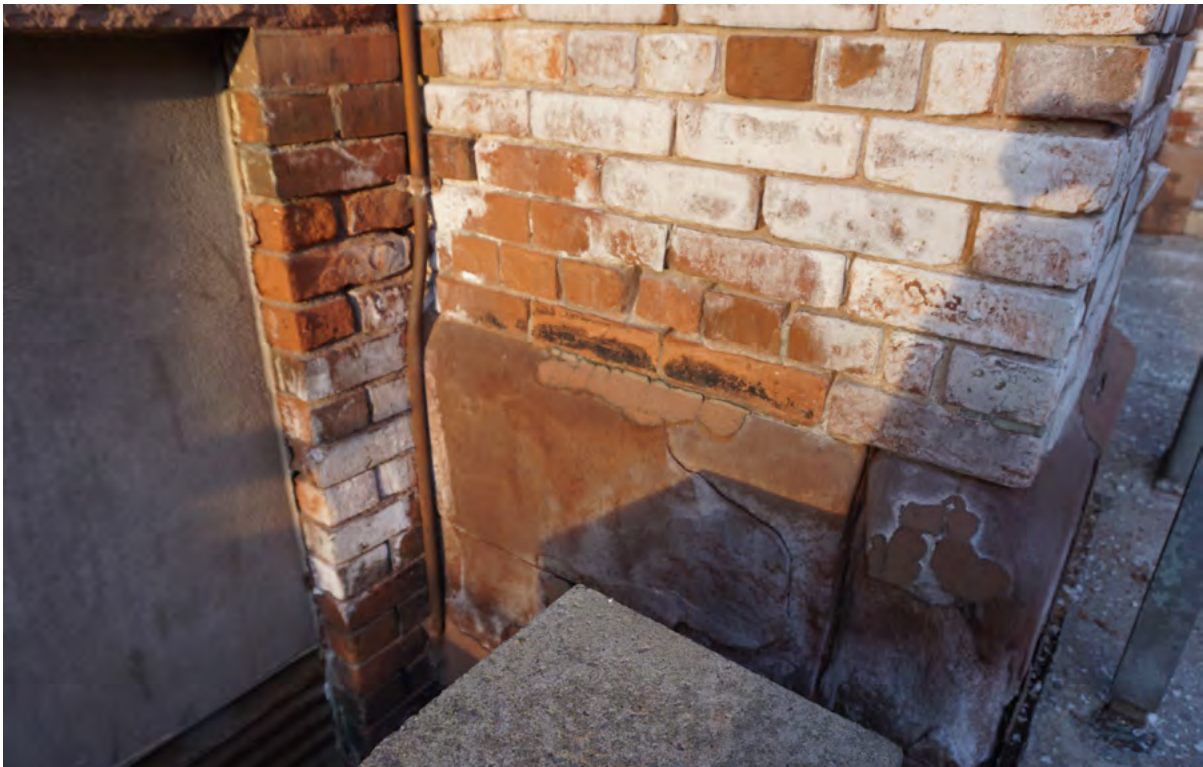
Link addition south elevation, stone and brickwork in an advanced state of deterioration (ERA, 2022)
