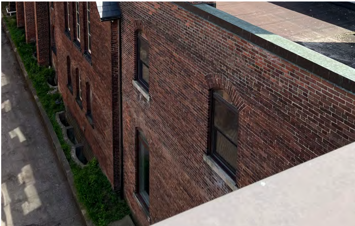
Link addition north elevation (foreground), replacement and infill of original windows in largely single plane simple brick facade (ERA, 2022)
