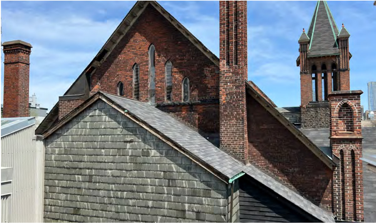
View from the 1889 Chapel/1913 Sunday School roof showing the variety of materials used on the Sanctuary building and structures at roof level, including the redundant brick chimneys (ERA, 2022)
