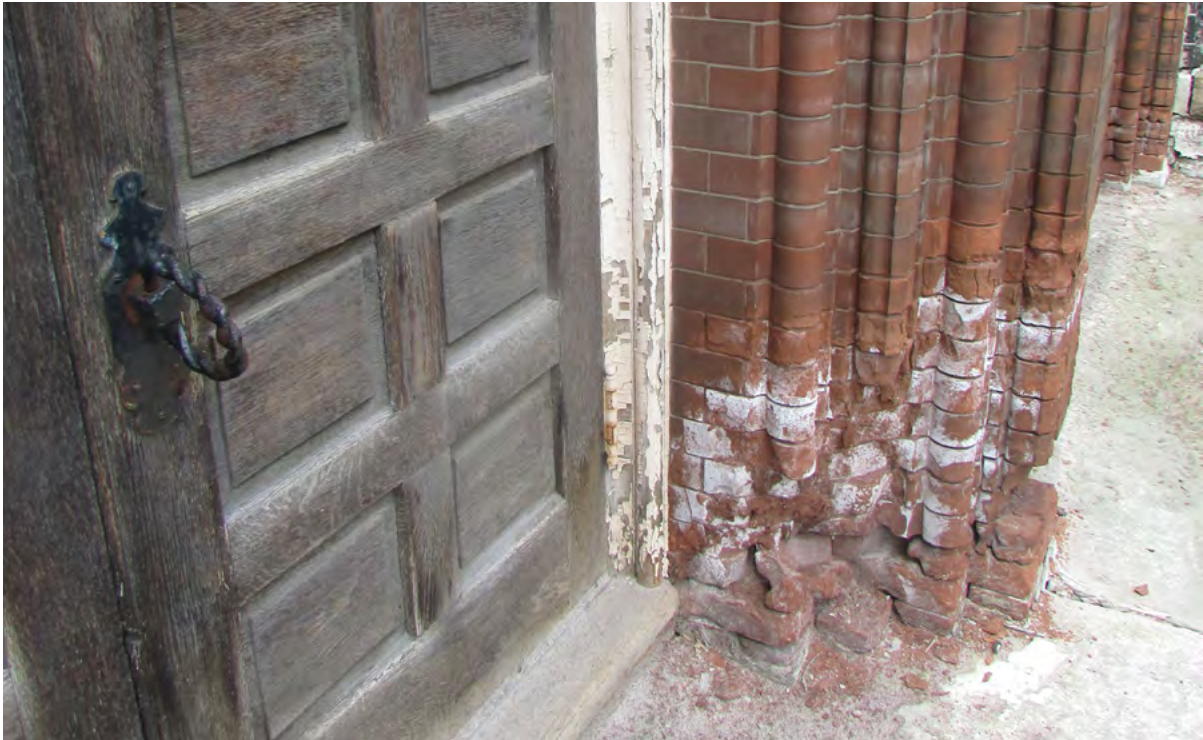
Sanctuary building east elevation, decorative brickwork in an advanced state of disrepair (ERA, 2022)
