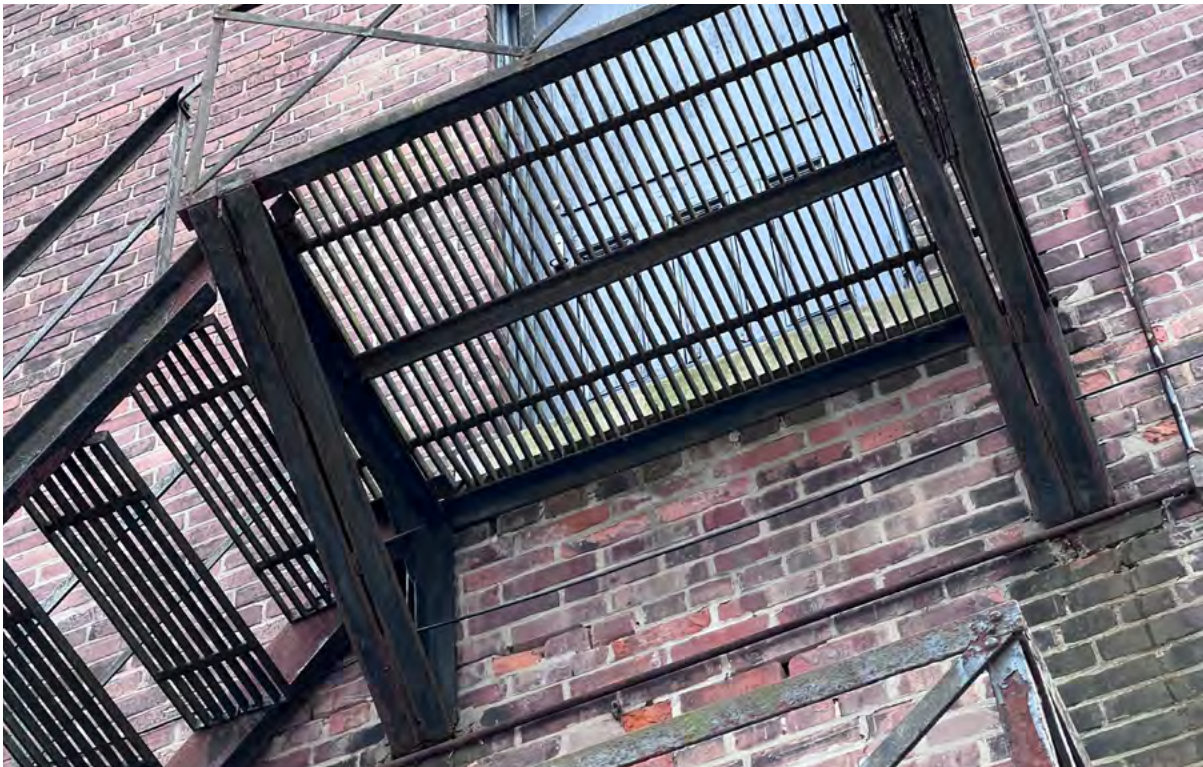
1889 Chapel/1913 Sunday School north elevation, stepped cracking and staining at exterior stair (ERA, 2022)
