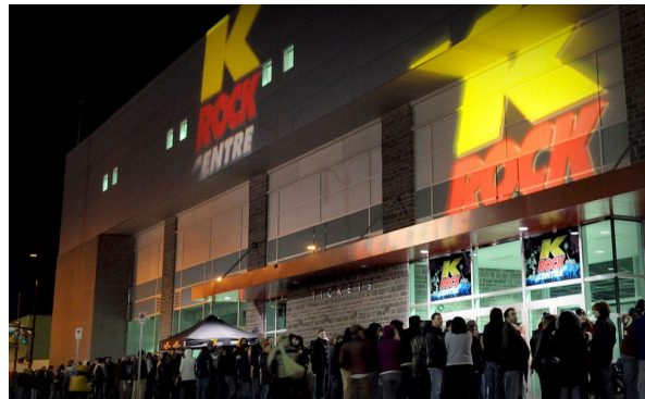
K-ROCK Centre Kingston, ON
