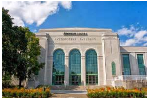
Allstream Centre, Toronto, ON
