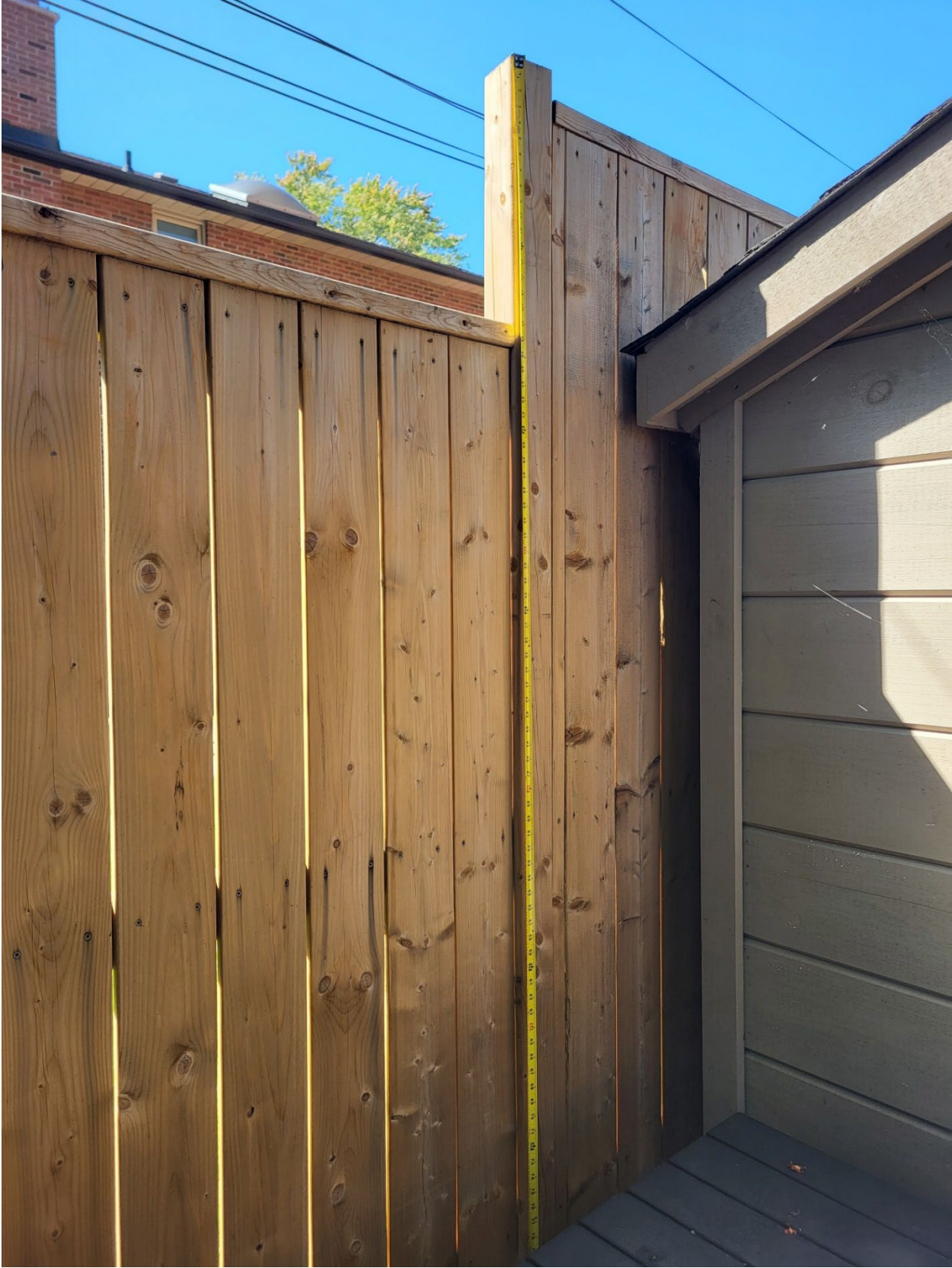
(West side of fence along shed measurement 2.5m)
