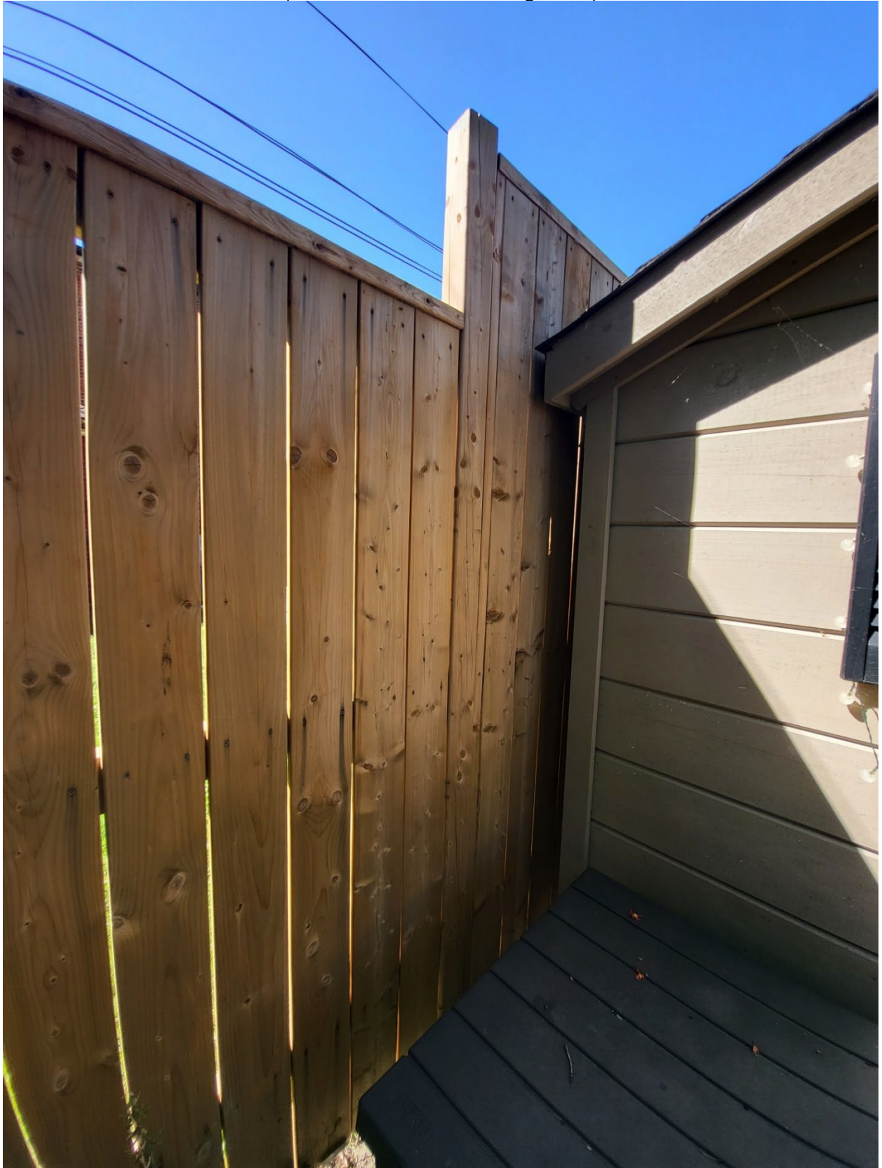
(West side of fence along shed)
