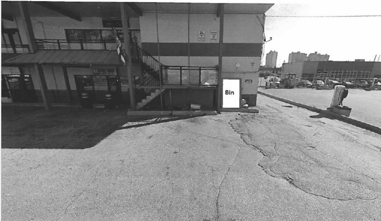
Attachment 2 - Photo of clothing drop box location
