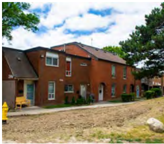
Existing low rise buildings in Jane Finch (townhouses)
