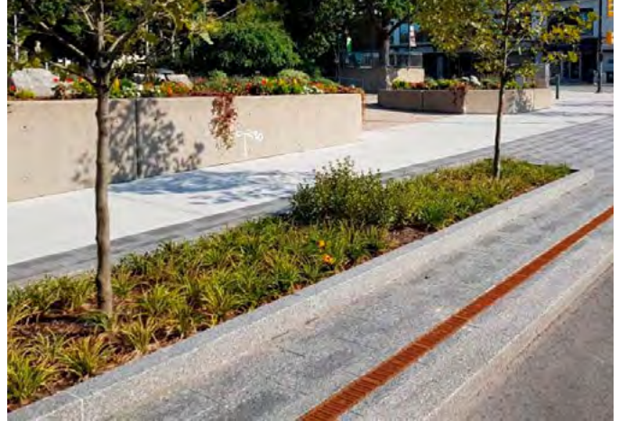
Integration of rain gardens into streetscape on Lakeshore Road (Photo from Brook McIlroy)
