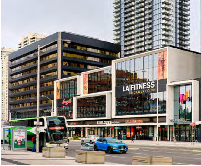
Yonge-Sheppard Centre features taller storey heights to accommodate non-residential uses such as supermarkets, restaurants, gyms, and retail (Photo from Archilovers)
