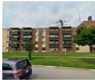
Existing low rise apartments that are typically 'slab' type buildings
