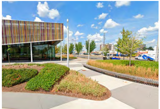
Paving, landscaping, and canopies provide comfortable spaces - Albion Library, Toronto (Google Maps)
