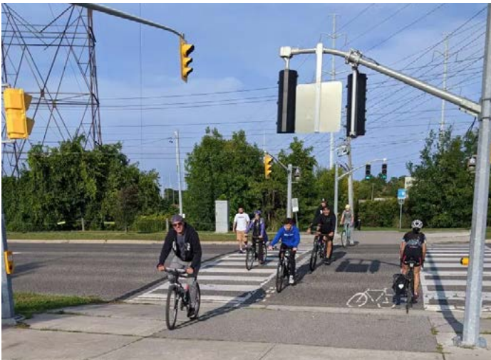
Figure 117. Signalized crossing for pedestrians and cyclists in Scarborough, along the Gattineau Hydro Corridor (Cycle Toronto)
