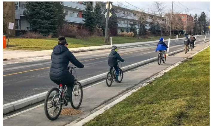
Figure 140. Concrete buffer between cyclists and vehicular traffic may be a quick build solution to create separation, Toronto (City of Toronto)
