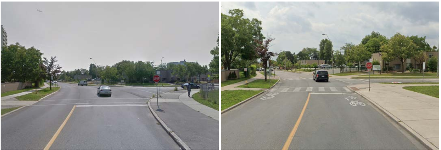
Figure 130. Example of intersection in the study area (Driftwood Ave and Yorkwood Gt) that has experienced a curb radii reduction and parking markings (left: before, right: after)
