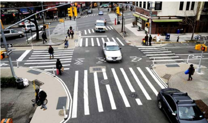
Figure 128. Reduced curb radii can help reduce pedestrian and cyclist crossing distances (NACTO)
