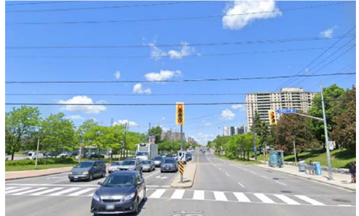
Figure 112. Jane Street at Finch has a crossing distance of over 30m for pedestrians, 2019, before LRT construction (Google Maps)
