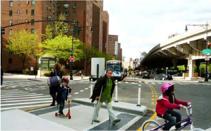
Figure 115. Safety island in New York is an example of a pedestrian and cycling safety measure (NACTO)
