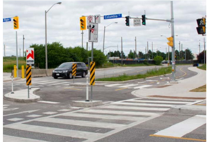
Figure 116. Example of a protected intersection and safer crossing experience at Murray Ross Parkway and Columbia Gate (Perkins&Will)
