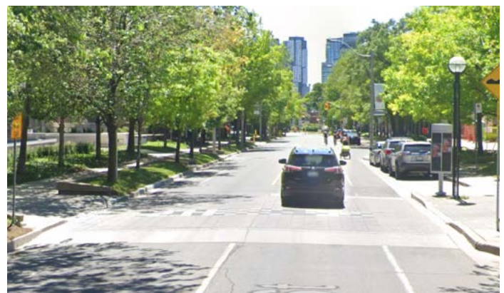
Figure 120. Example of raised crosswalk, unique paving, and signage to force vehicles to slow down – University of Toronto, St. George Street (Google Maps)
