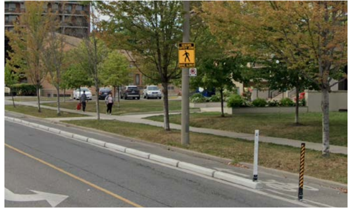
Figure 122. Example of safety improvements on an arterial - cycling buffer (concrete buffer and bollards) and senior safety zone signage, Thorncliffe Park, Toronto (Google Maps)
