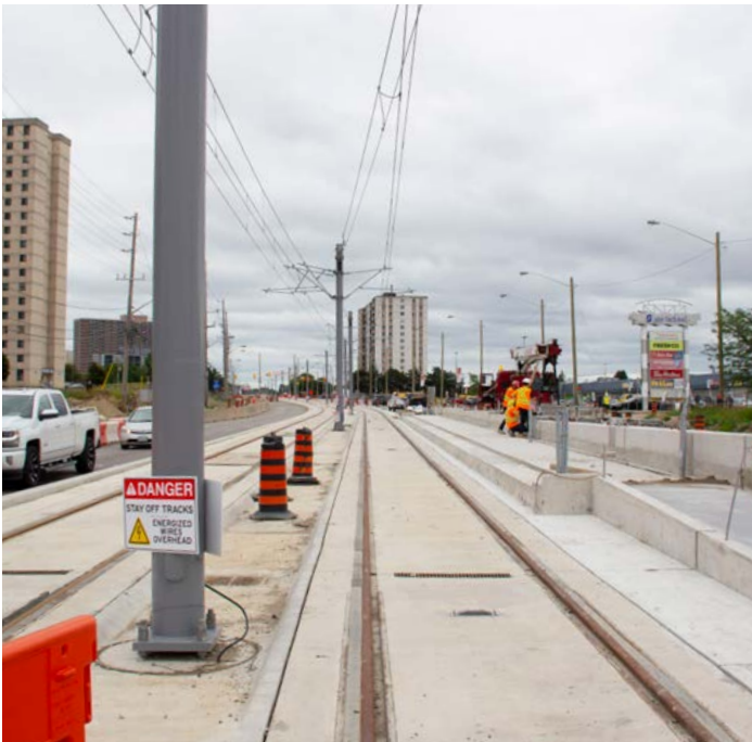
Figure 110. The in-progress Finch West LRT construction (Perkins&Will)
