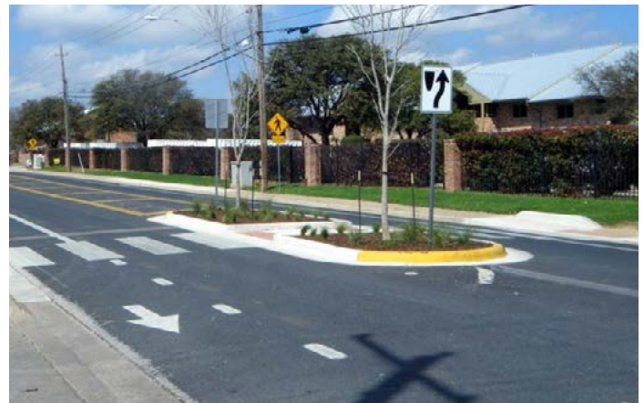
Figure 118. Safety islands limit pedestrian exposure in an intersection and help people feel less vulnerable in the street (NACTO)
