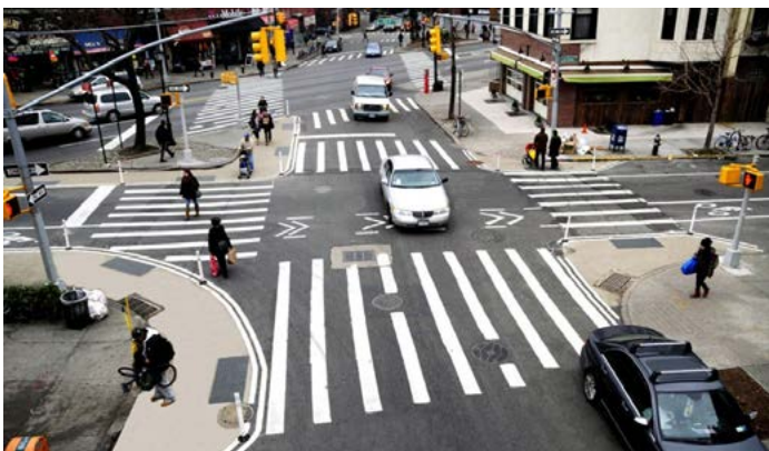
Figure 129. Reduced curb radii can help reduce pedestrian and cyclist crossing distances (NACTO)
