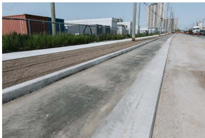
Figure 188. Cycle tracks under construction along Finch provide a curbed buffer between cycling infrastructure and the roadway (@FinchWestLRT on X.com)
