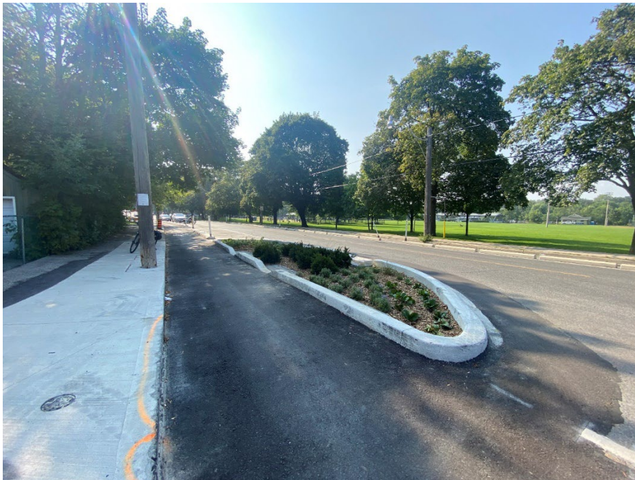
Figure 43: In 2023, Transportation Services updated Dundas Street East between Greenwood Avenue and Alton Street, including a planted median and poured-in-place concrete separating the cycle track and motor vehicle parking and travel lanes. If approved, Dundas Street East between Broadview Ave and West Ave and between Logan Ave and Pape Ave would have a similar treatment.
