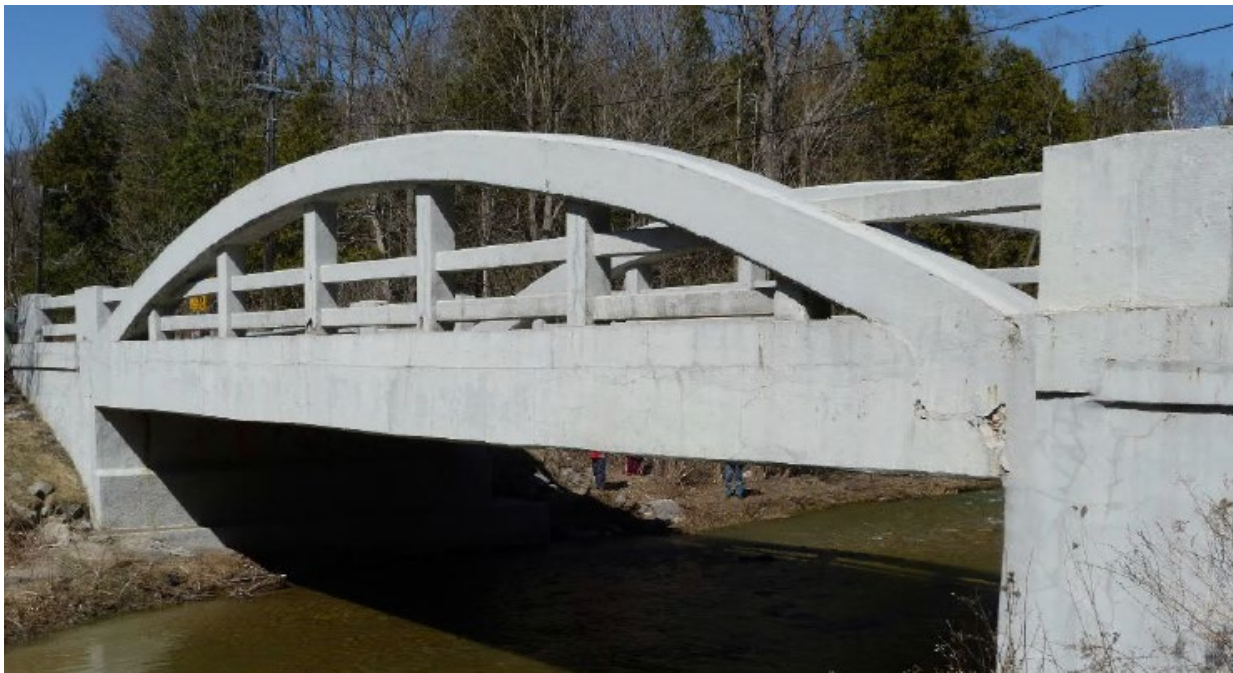
View of Maxwell's Bridge
