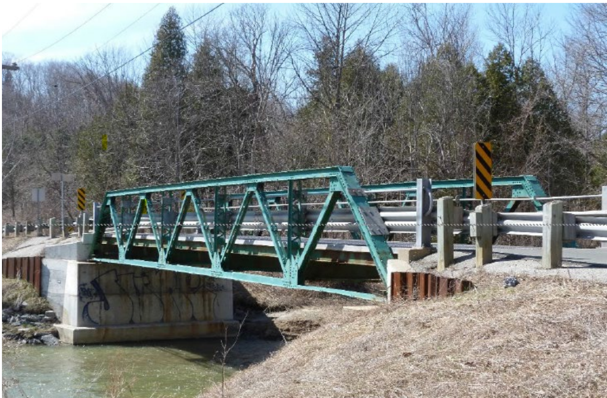
View of Stott's Bridge
