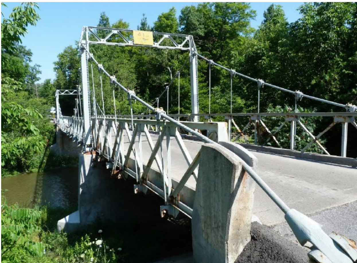
View of Sewells Road Suspension Bridge
