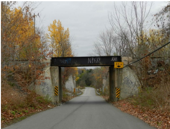
View of CP Rail Bridge over Sewells Road
