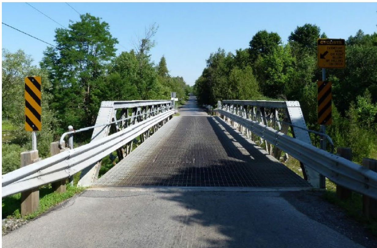
View of Hillside Bridge
