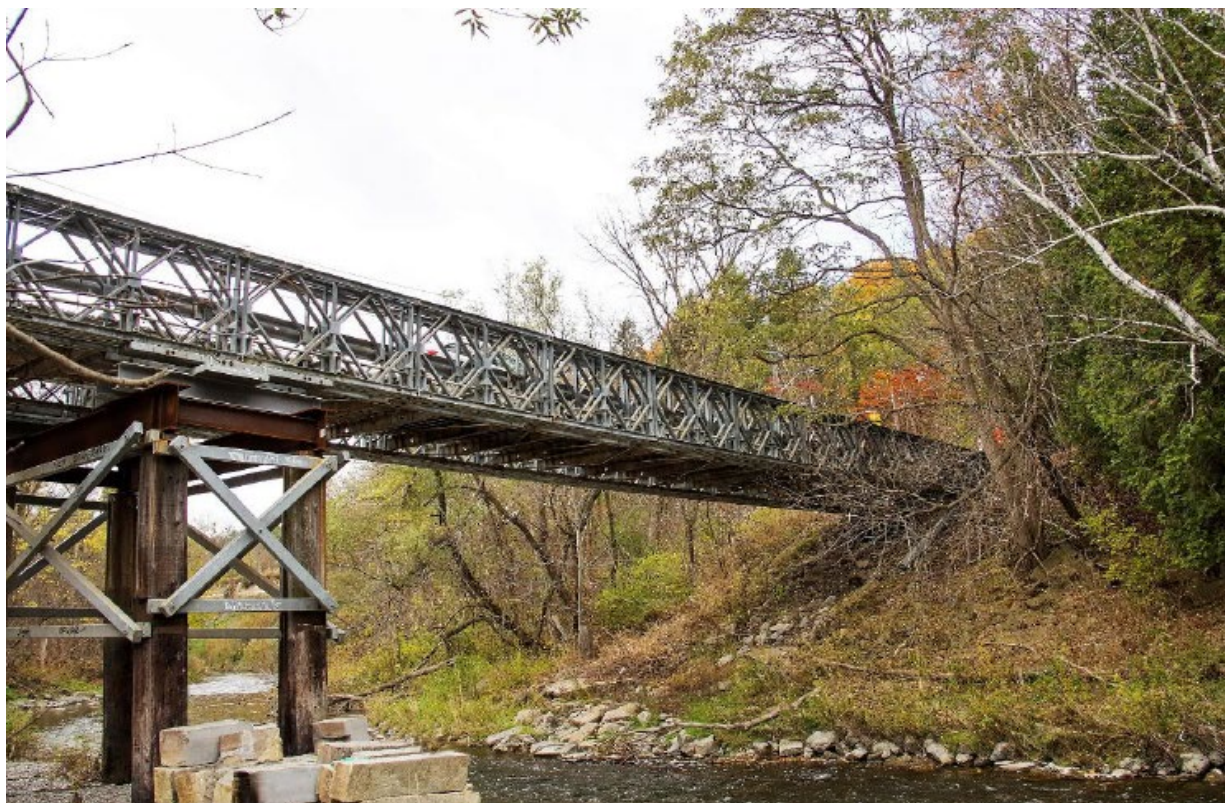
View of Milne Bailey Bridge
