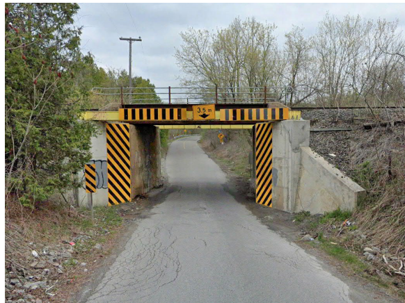
View of CP Rail Bridge over Meadowvale Road
