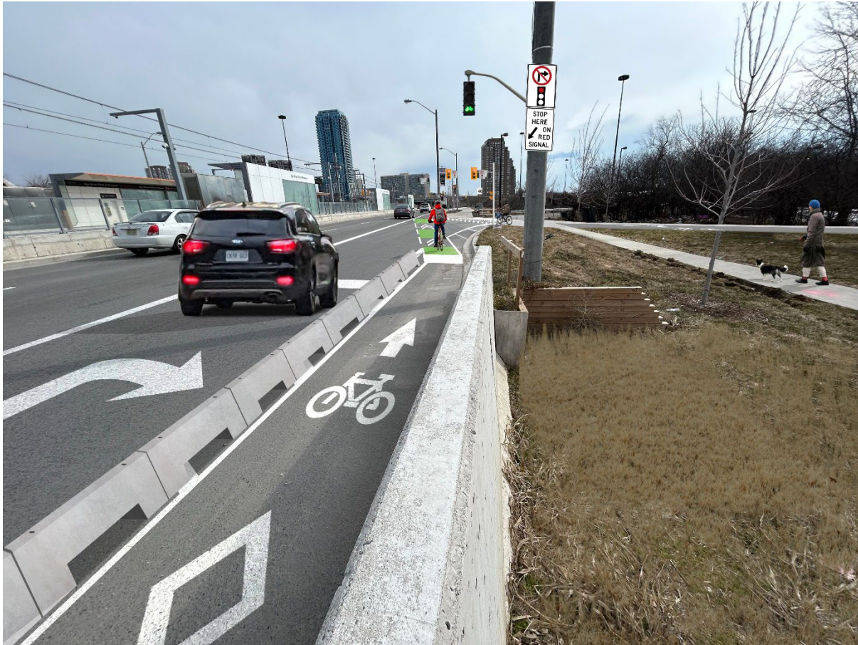
Figure 4: An artist rendering of the westbound to southbound Don Valley Parkway ramp. The proposed design includes a new traffic signal at the ramp with barriers to separate the bike lane and the motor vehicle lane.
