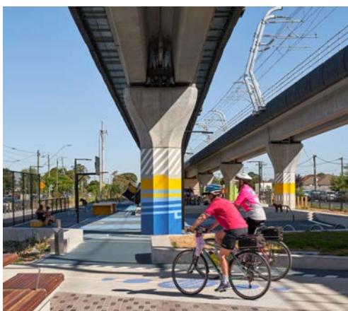
Image 10: The Caulfield to Dandenong Level Crossing Removal project, Melbourne, Australia.
