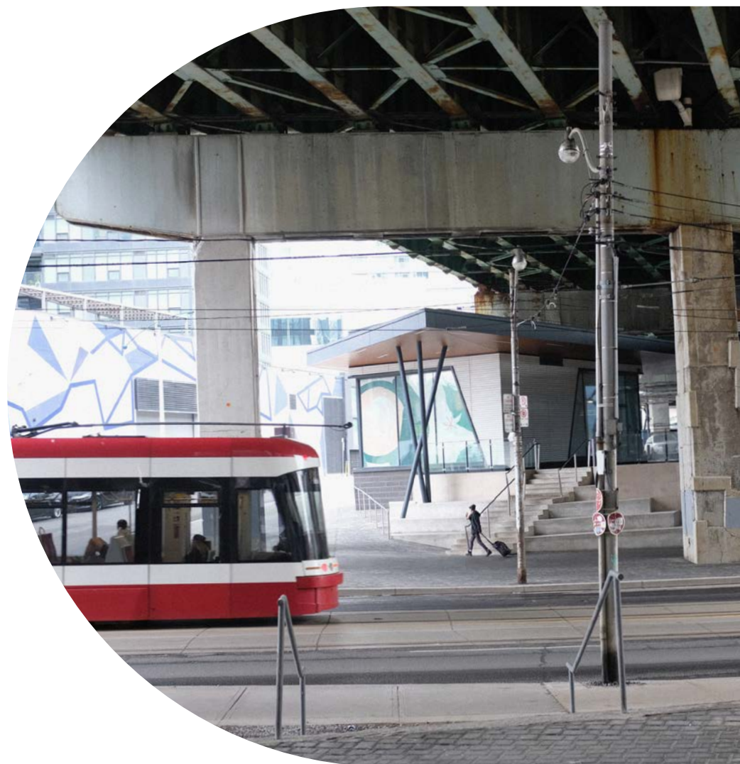
Image 35: The current condition of the Bathurst Street crossing under the Gardiner Expressway. Precise crossing location to be confirmed through further study. Already a highly-trafficked desire line, formalizing this crossing will ensure safety of all users.
