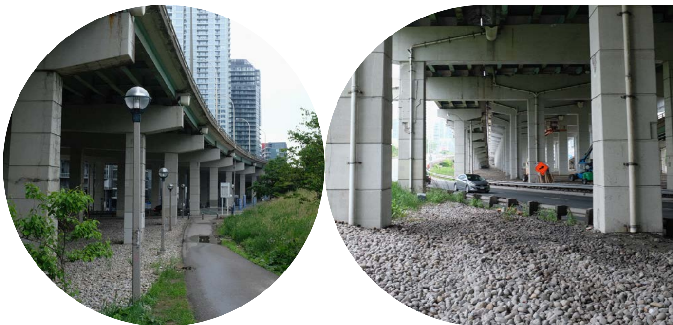
Image 36: Left: View looking west of the Dan Leckie-Lake Shore Triangle and Terry Fox Miracle Mile trail. Right: View looking east toward the Spadina off-ramp and the Dan Leckie-Lake Shore Triangle.
