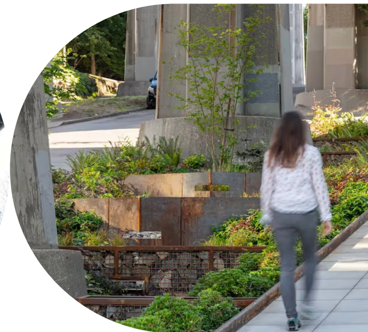
Image 41: Stepped blue-green medians supporting urban vegetation below the Aurora Bridge in Seattle, WA.
