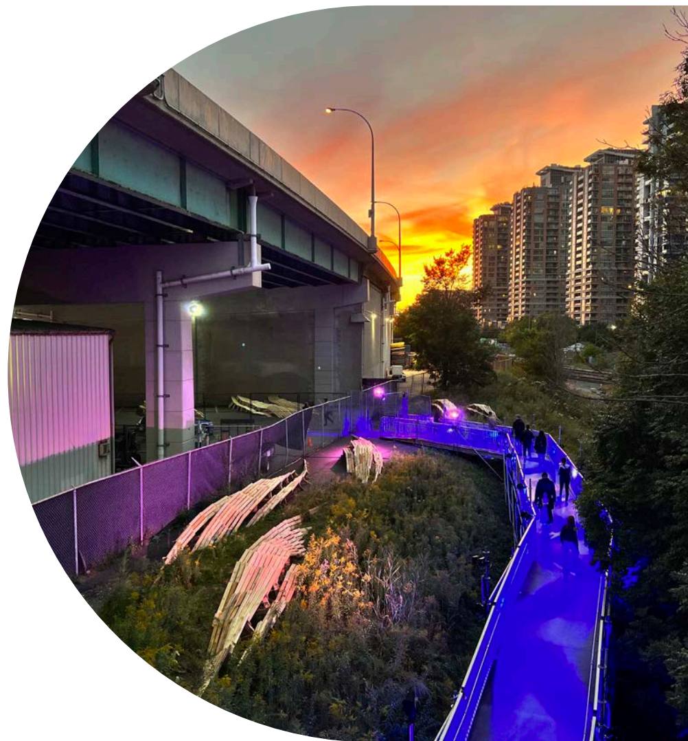
Image 31: View looking west from Strachan Avenue. Pictured temporary Strachan Gate Connection temporarily installed for October 2021 and 2022, demonstrating a potential link between The Bentway and Exhibition Place.
