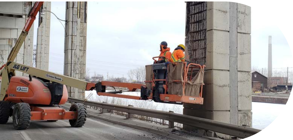
Image 46: Maintenance operations on a bent under the Gardiner Expressway.
