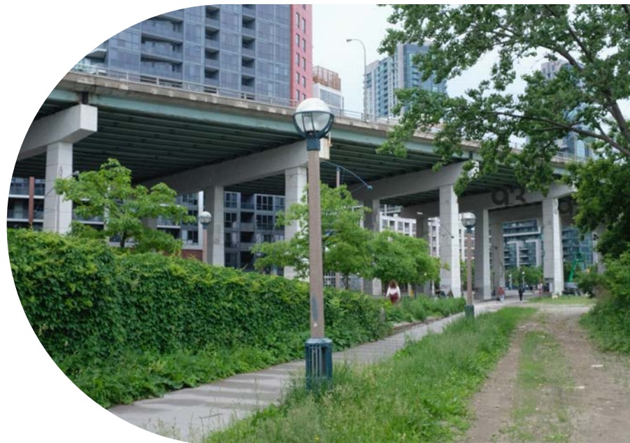
Image 34: View southwest toward The Bentway Phase 1 site from the future Lower Garrison Creek Park connection.
