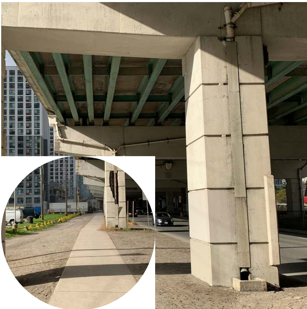
Image 42: View of the existing pedestrian path south of Lake Shore Blvd West, below the Gardiner Expressway, looking west
