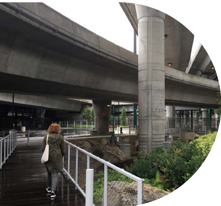
Image 39: Rainwater management landscape at Infra-Space 1 in Boston treats water diverted from the elevated highway above.
