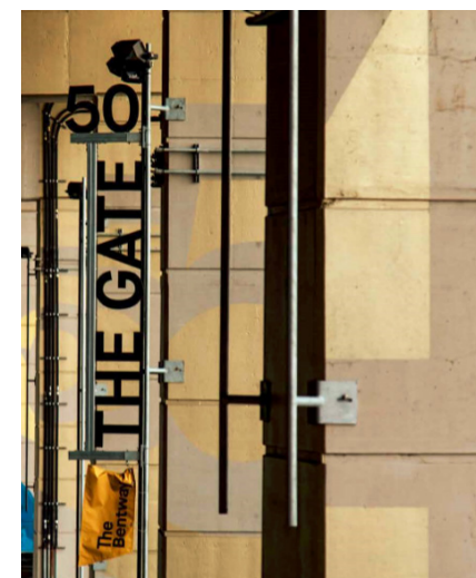
Image 22: (above) An example of an effective bent-mounted floodlight system from The Bentway Phase 1 site.
