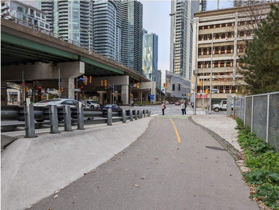
Figure 16: Obstructed sight lines exist between eastbound people cycling and eastbound right-turning drivers increases chance of collisions. The multi-use trail is not within the view of drivers' side-view mirrors.
