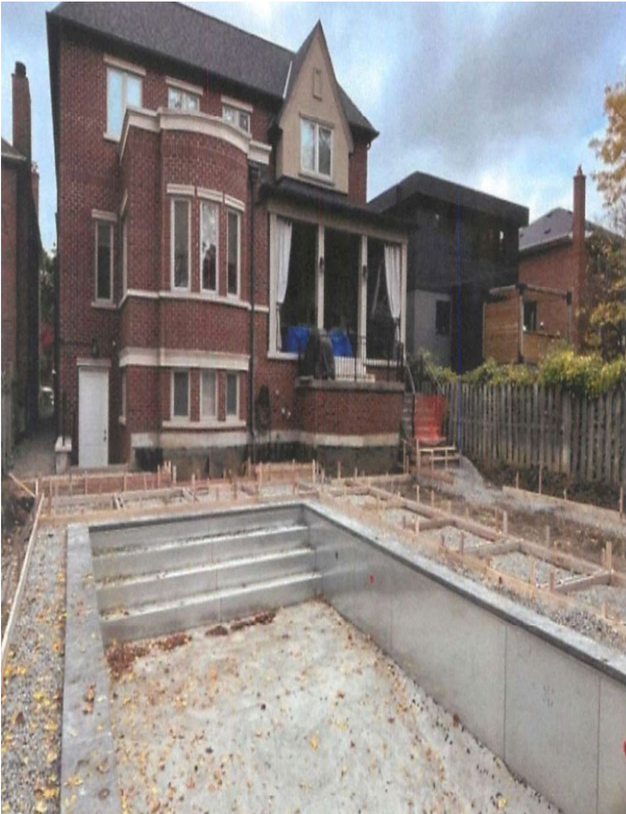
Attachment 4: Applicants Photo – Exterior Walkout/Basement Door & Pool
