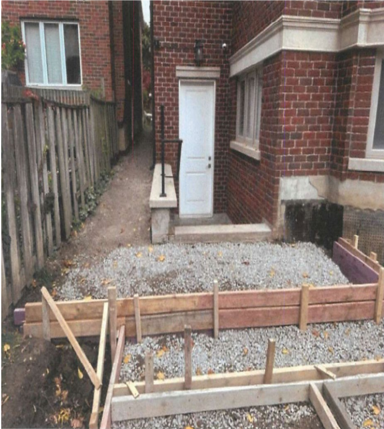
Attachment 3: Applicants Photo – Exterior Walkout/Basement Door
