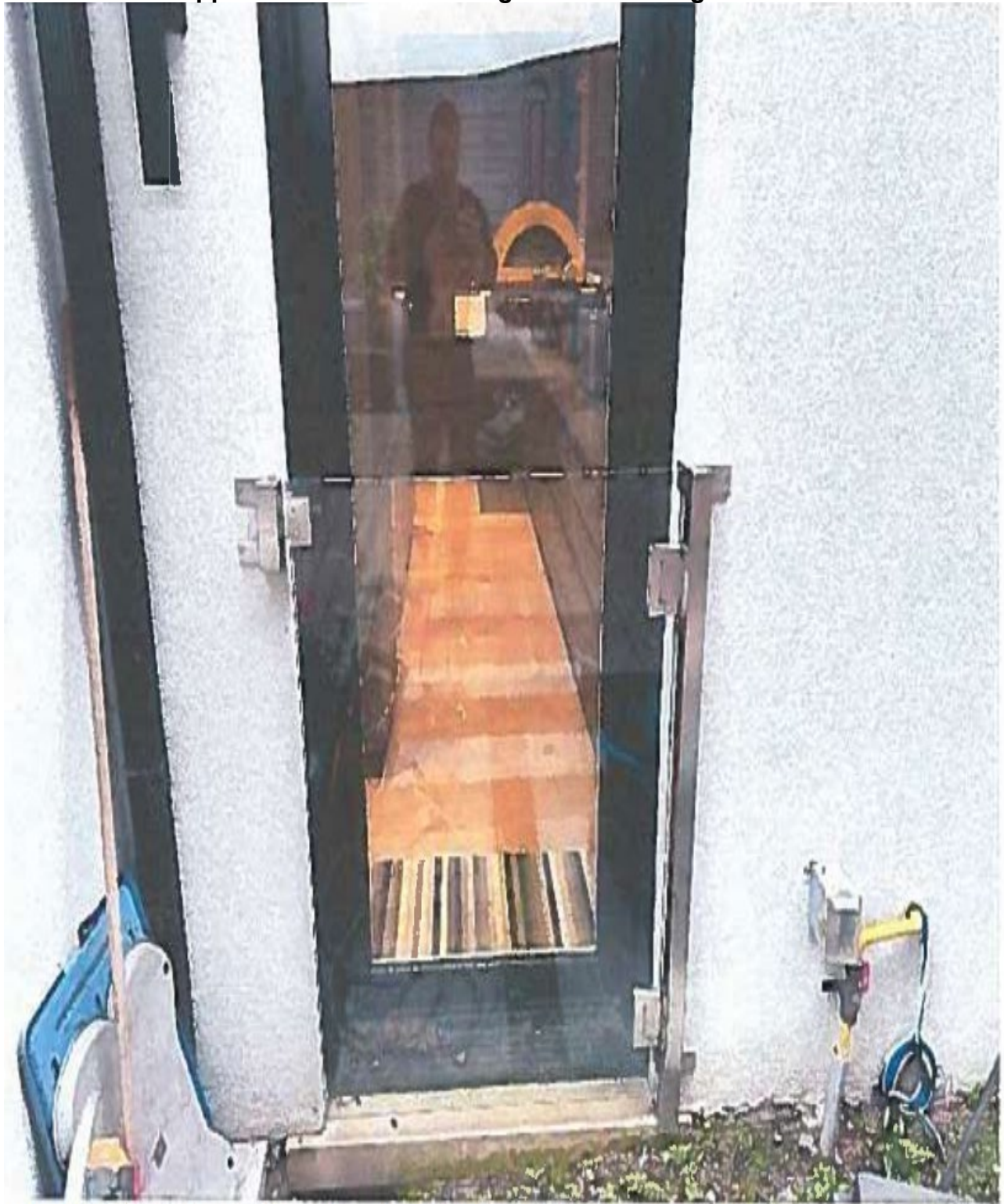
Figure 5: Glass door #1 with self-closing, self-locking mechanism
