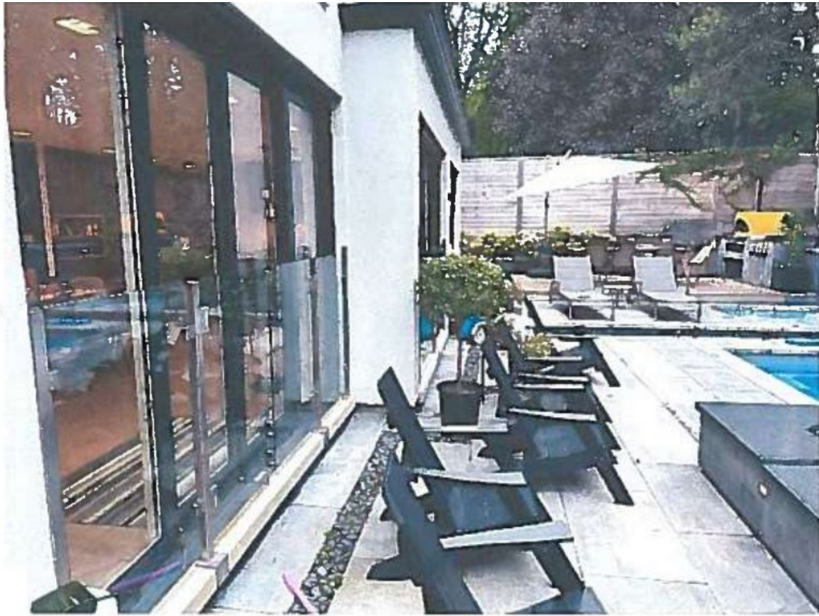
Figure 3: Glass door #3 at rear of house with self-closing, self-locking gate
