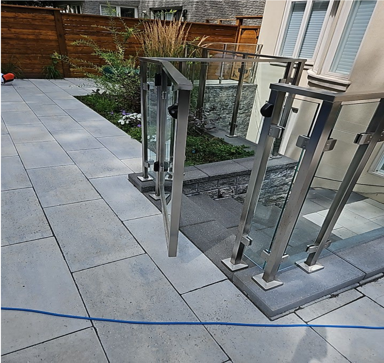
Attachment 5: Municipal Standards Officer's Photo - 115 Munro Boulevard - Existing pool Enclosure. – Pool Gate.
