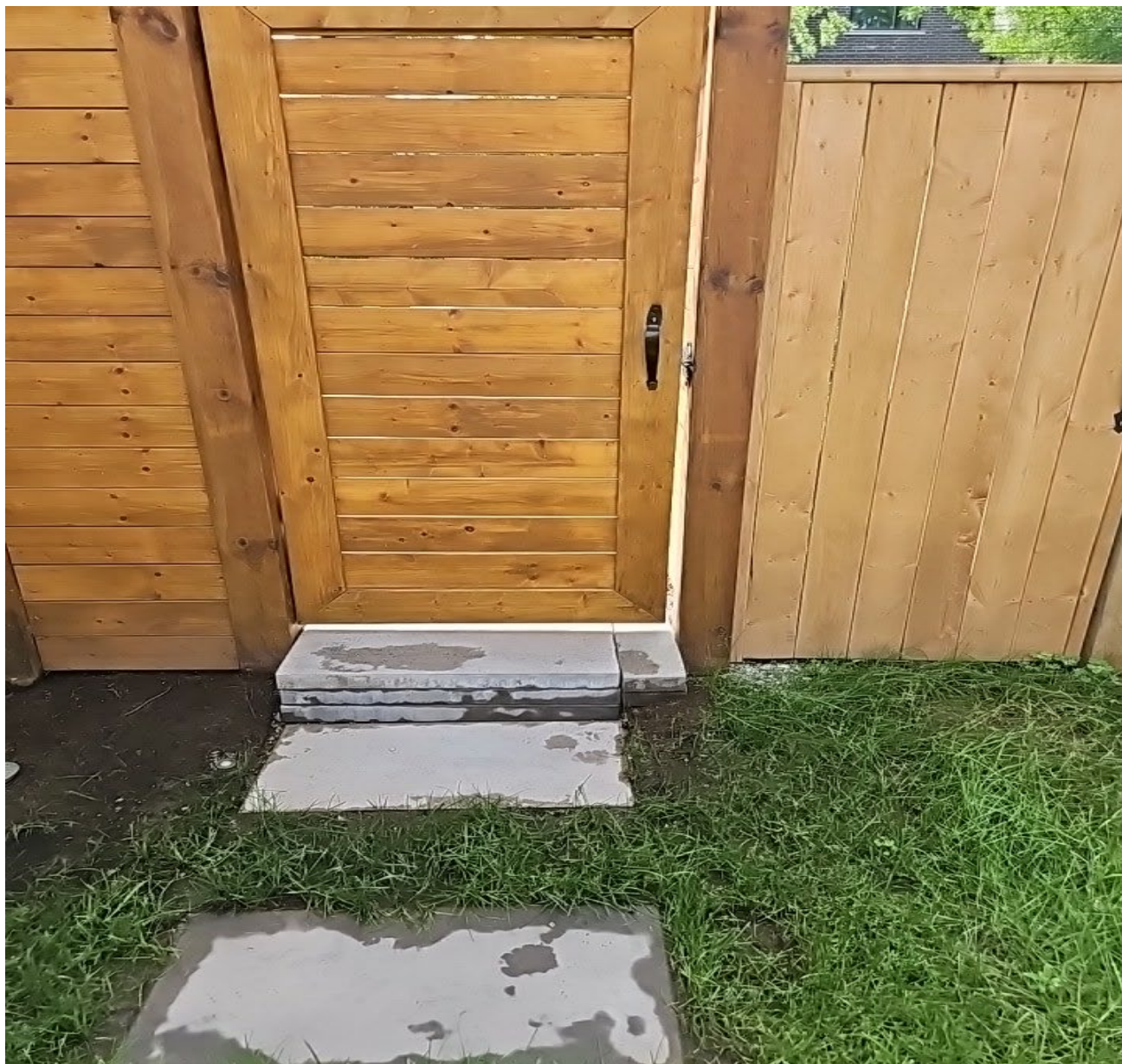
Attachment 4: Municipal Standards Officer's Photo - 115 Munro Boulevard - Existing Pool Enclosure. – Pool Gate - Side Yard
