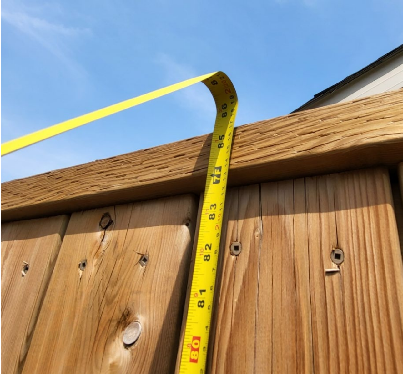
Attachment 5: Municipal Standards Officer's Photo – 311 Patricia - Existing pool Enclosure. - Fence Height.
