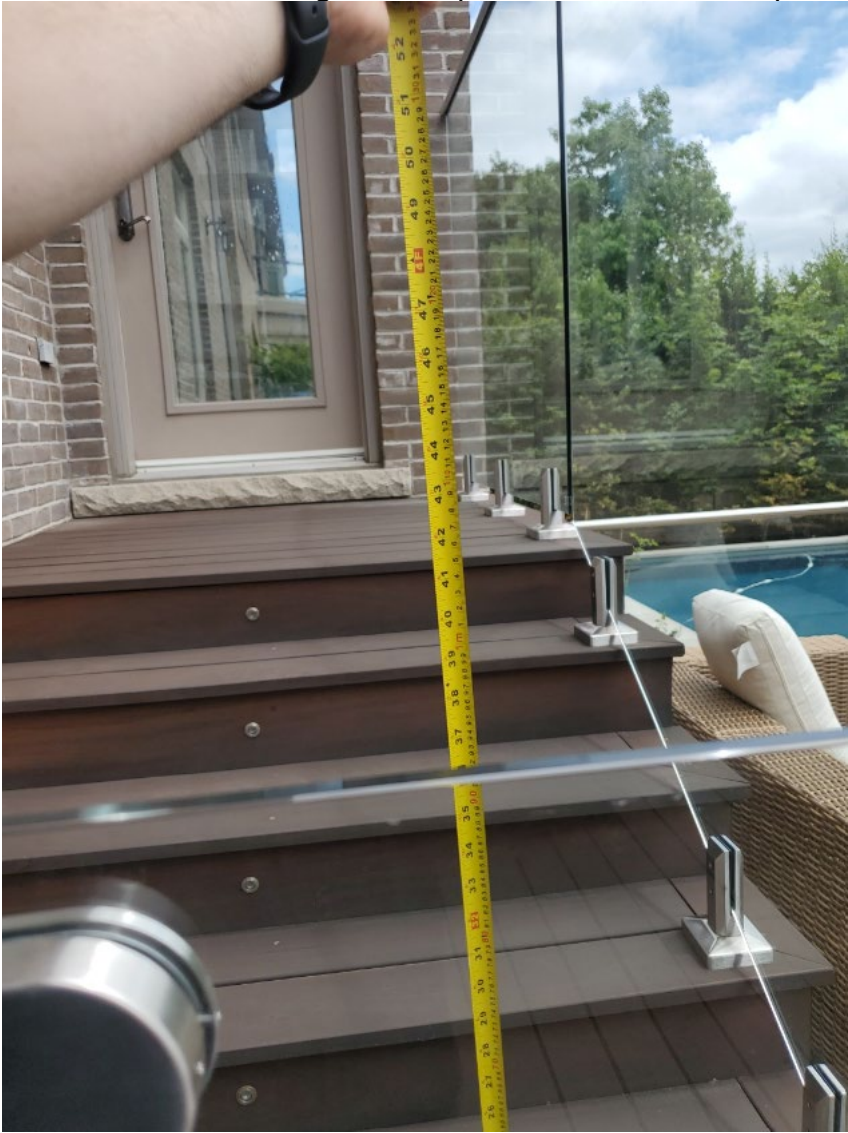
Attachment 4: The height of the pool enclosure from top of stair raiser.
