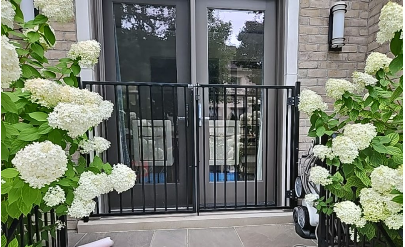
Attachment 3: The staircase from the deck forming part of the pool enclosure.
