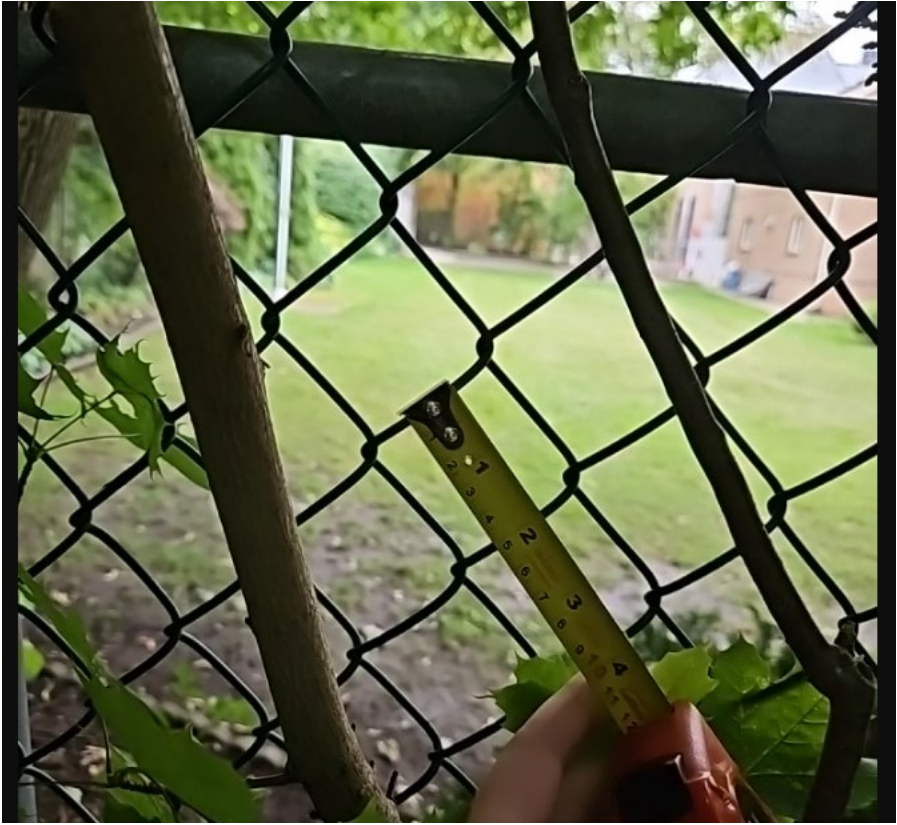
Attachment 2: Municipal Standards Officer's Photo 53 Yorkminster Road - West side of the existing pool enclosure.
