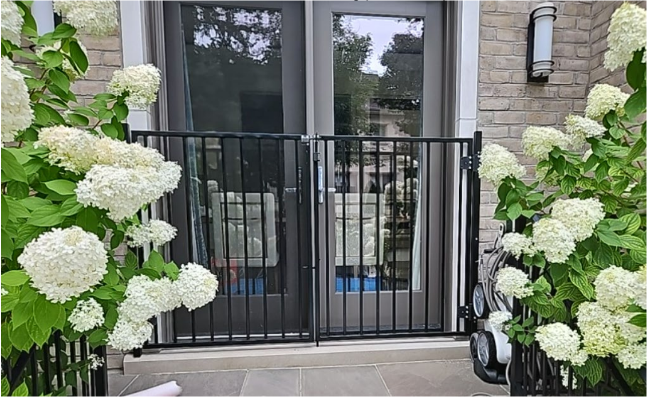
Attachment 3: The staircase from the deck forming part of the pool enclosure.
