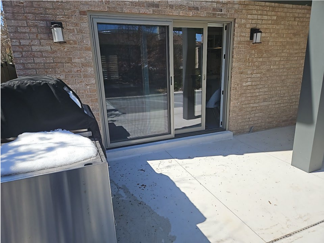
Attachment 2: Municipal Standards Officer's Photo - 51 Tanbark Cres - Rear Yard dwelling access to pool area.
