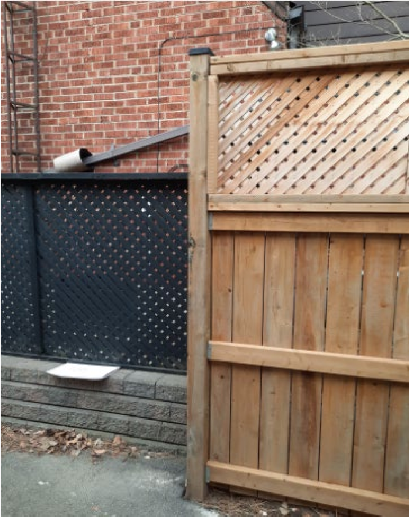
Attachment 3: Municipal Standards Officer's Photo 79 Yorkview Drive – Side Yard
