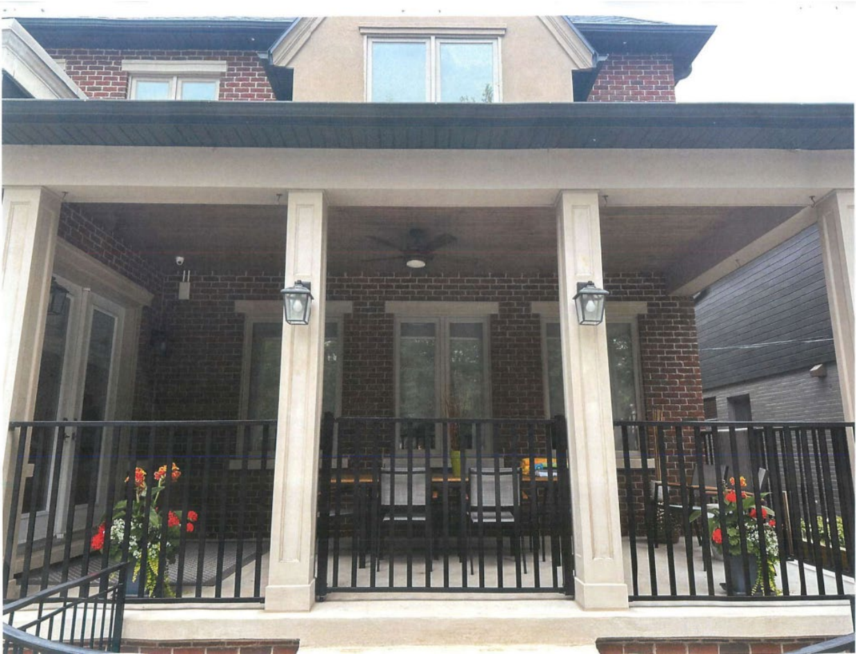
Attachment 2: Applicant Photo - Rear Balcony Guard
