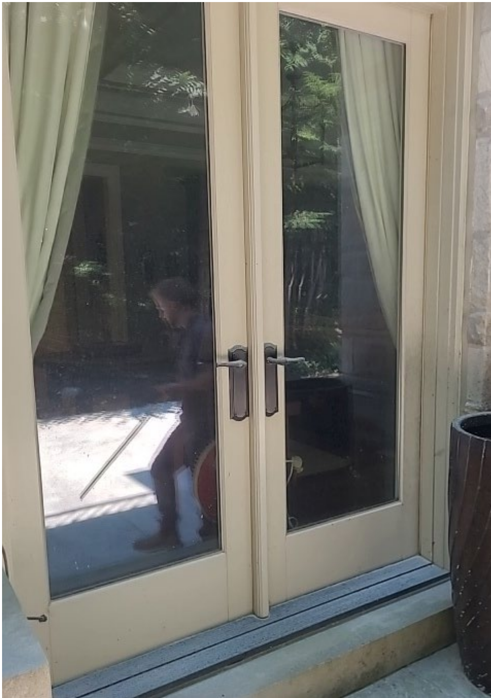
Attachment 3: North most patio doors of rear dwelling
