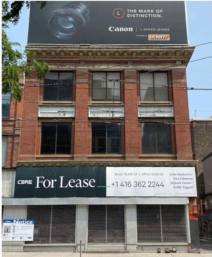
West (principal) elevation of 119 Church St
