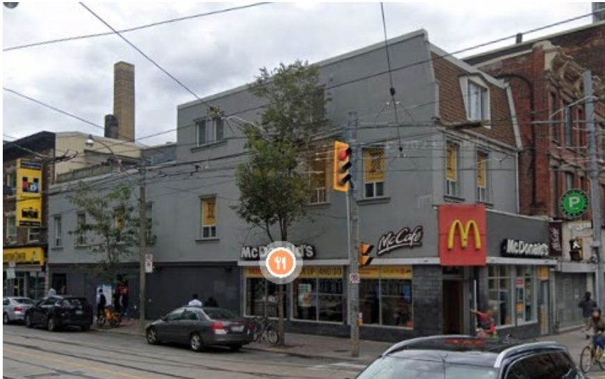
North and west elevations of 125-127 Church Street
