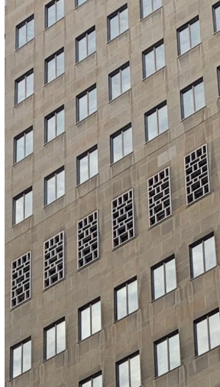
Images 29 and 30. At left, a current photo of the south elevation; at right, a detail of the south elevation showing the decorative metal grilles at the 13th storey, which also serve as a datum line for the building's pre-1966 vertical termination. (Heritage Planning, 2023)
