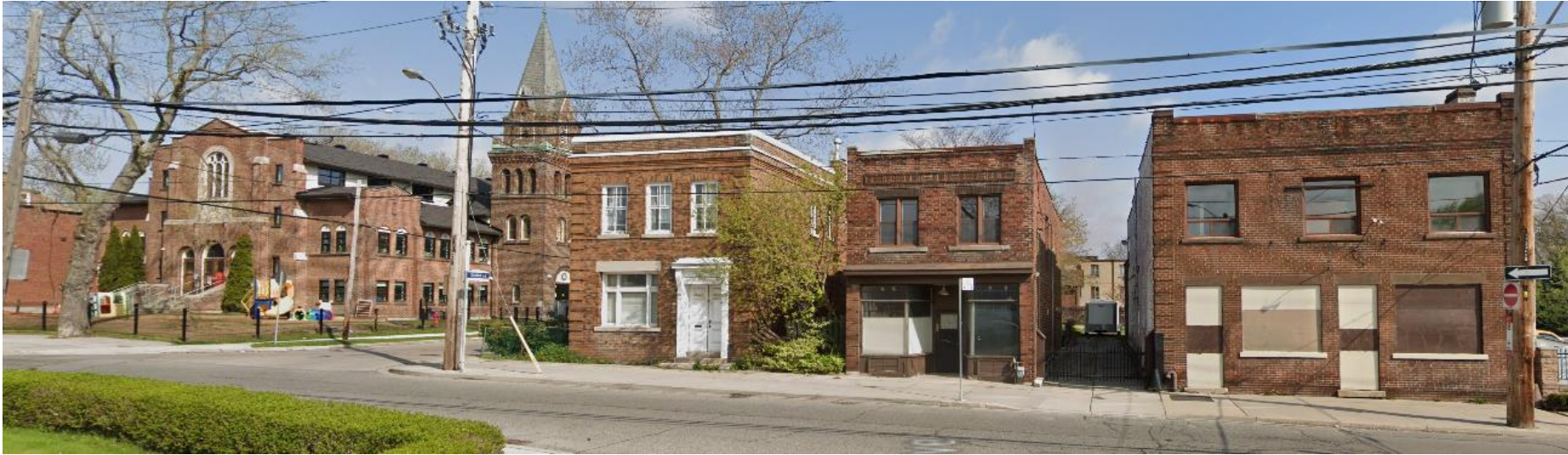
Wide view looking northwest towards the intersection of Mimico Avenue and Station Road (Google, April 2019).
