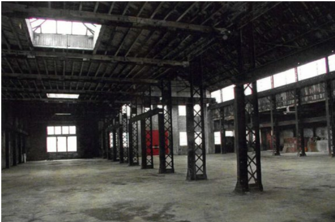
Figure 18. Interior view of the A. R. Williams Machinery Company Warehouse showing the volumes and features of the space including the steel support columns with cross braces and some of the skylights, c. 2005 (Heritage Planning)
