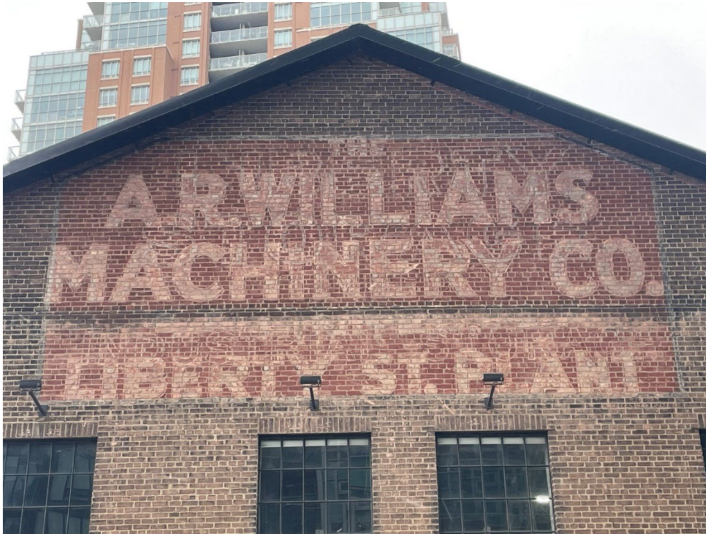
Figure 11. South elevation of the A. R. Williams Machinery Company Warehouse showing ghost signage for the "A.R. Williams Machinery Co. Liberty Street Plant, 2024 (Heritage Planning)
