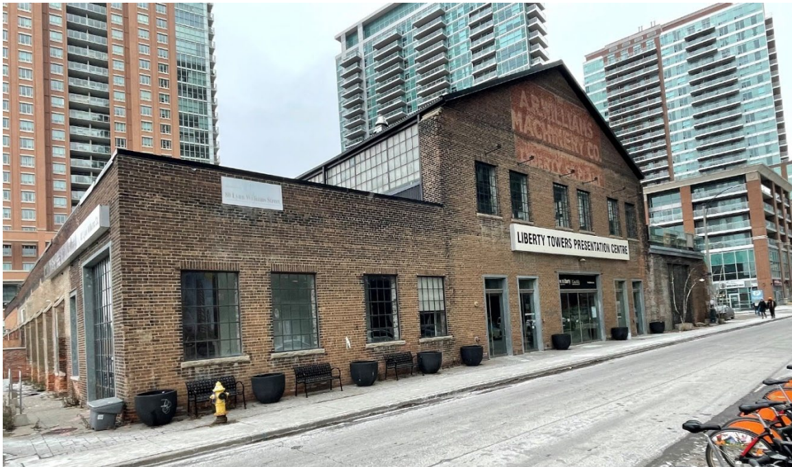
Figure 10. South elevation of the A. R. Williams Machinery Company Warehouse, 2024 (Heritage Planning)
