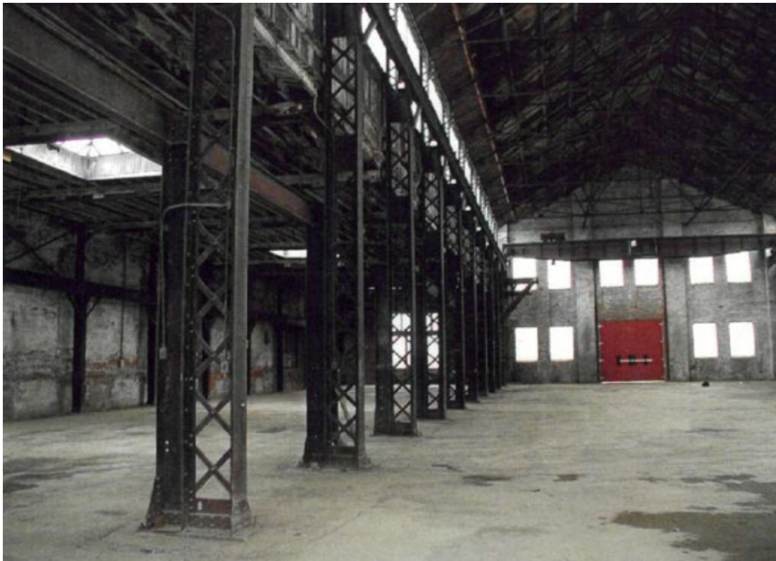
Figure 17. Interior view of the A. R. Williams Machinery Company Warehouse showing the volumes and features of the space including the steel support columns with cross braces, c. 2005 (Heritage Planning)
