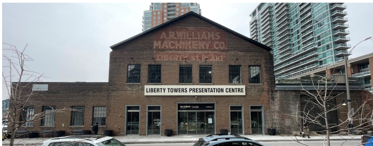
Figure 1. Main elevation (south) of subject property, facing onto Lynn Williams Street (Heritage Planning, 2024).
