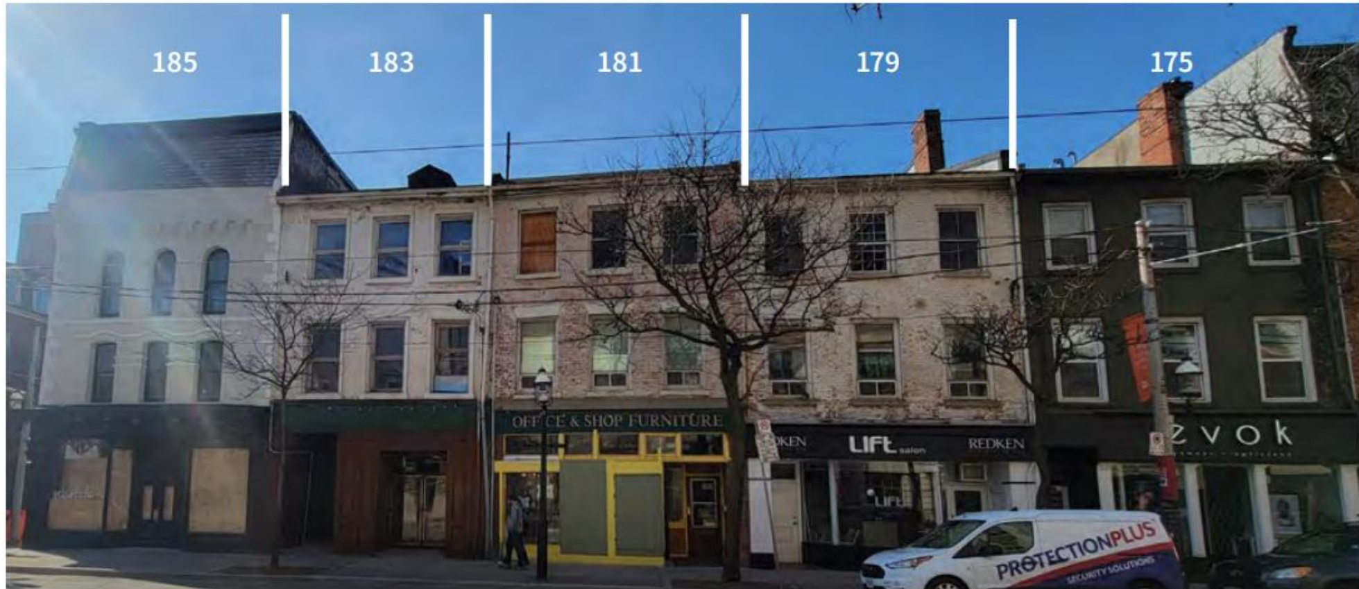
Contextual key map photograph showing the principal (north) elevations of the properties on King Street East. The street numbers of each property within the development site are indicated (ERA Architects Inc., 2022).
