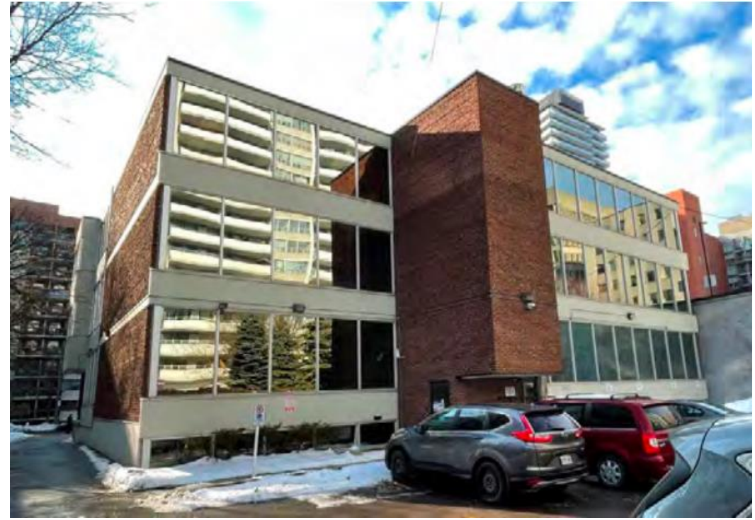
View of the north elevation showing the three-storey rear wing (Heritage Planning).
