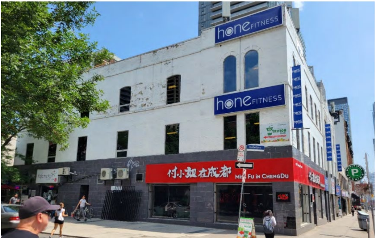
North Elevation of 625 Yonge Street (Source: HIA prepared by VG Architects Ltd.,).
