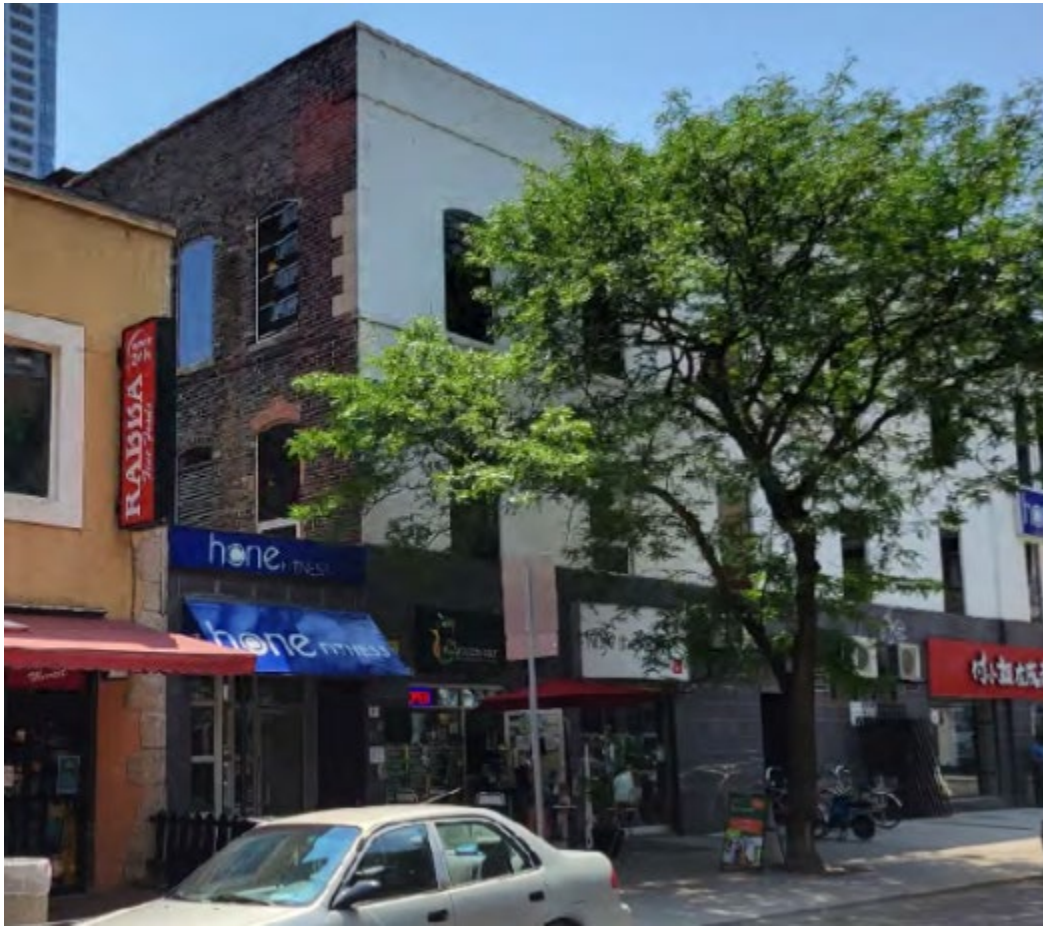
North and East Elevations of 625 Yonge Street (Source: HIA prepared by VG Architects Ltd.,).
