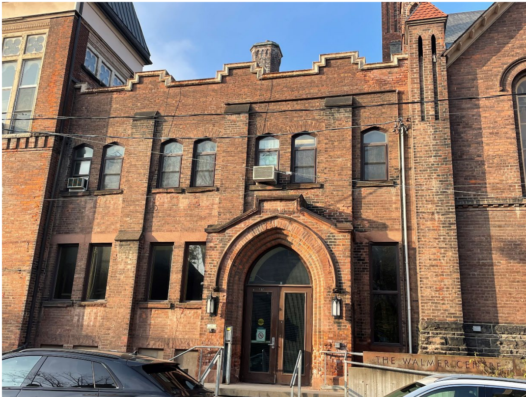
Front (south) elevation of the Memorial Building, 2022 (Heritage Planning)
