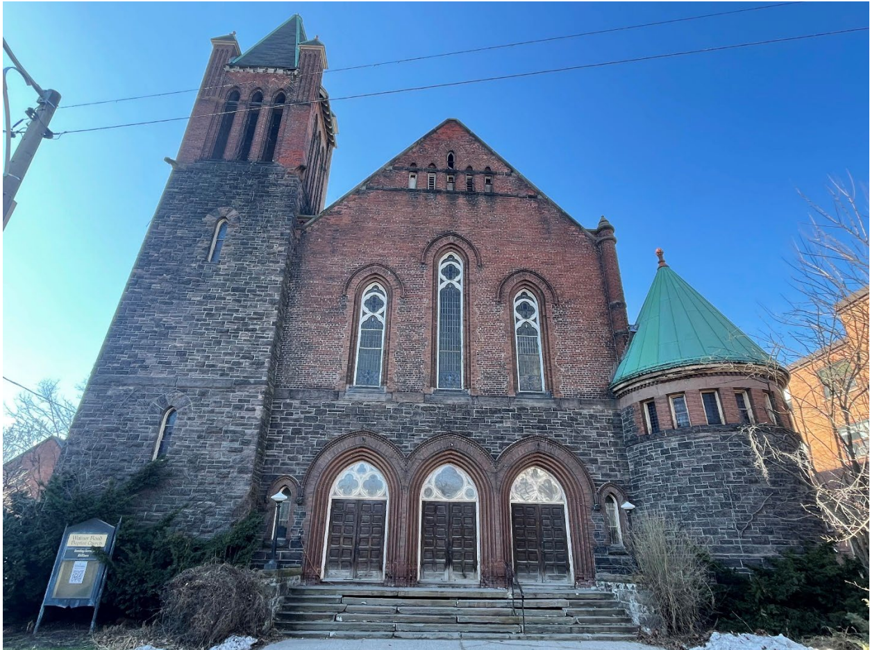
Front (east) elevation of the Sanctuary Building at 38 Walmer Road, 2023 (Heritage Planning)
