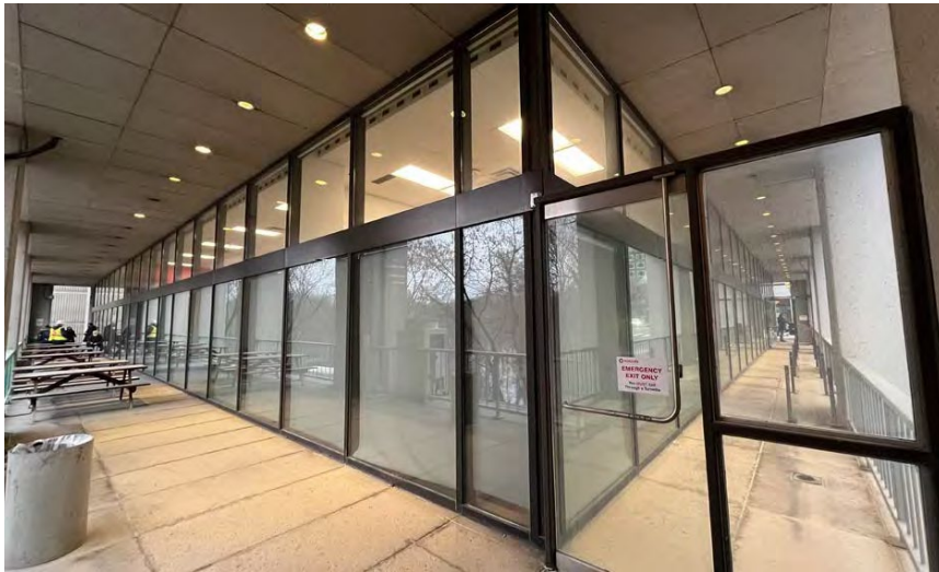
View of the pedestrian colonnade on the first level.
