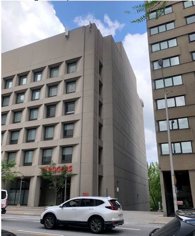
View of southwest corner of the building showing the east elevation with a predominant blank wall
