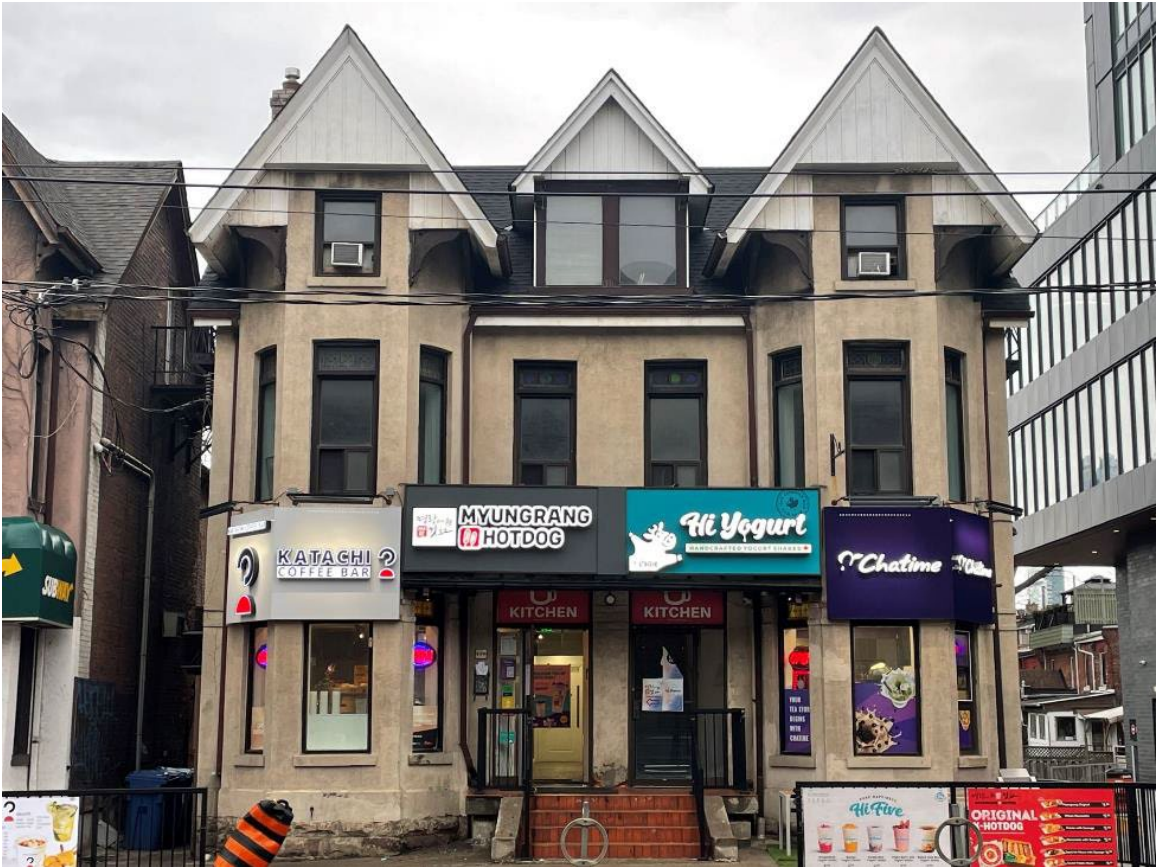
View of North/College Street Elevation of 199 College Street (Heritage Planning, 2022)
