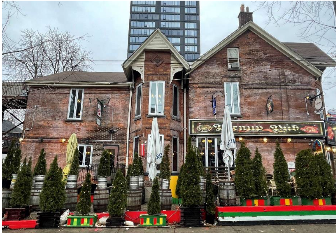
Secondary (east)/Henry Street elevation of 191 College Street. (Heritage Planning, 2022)
