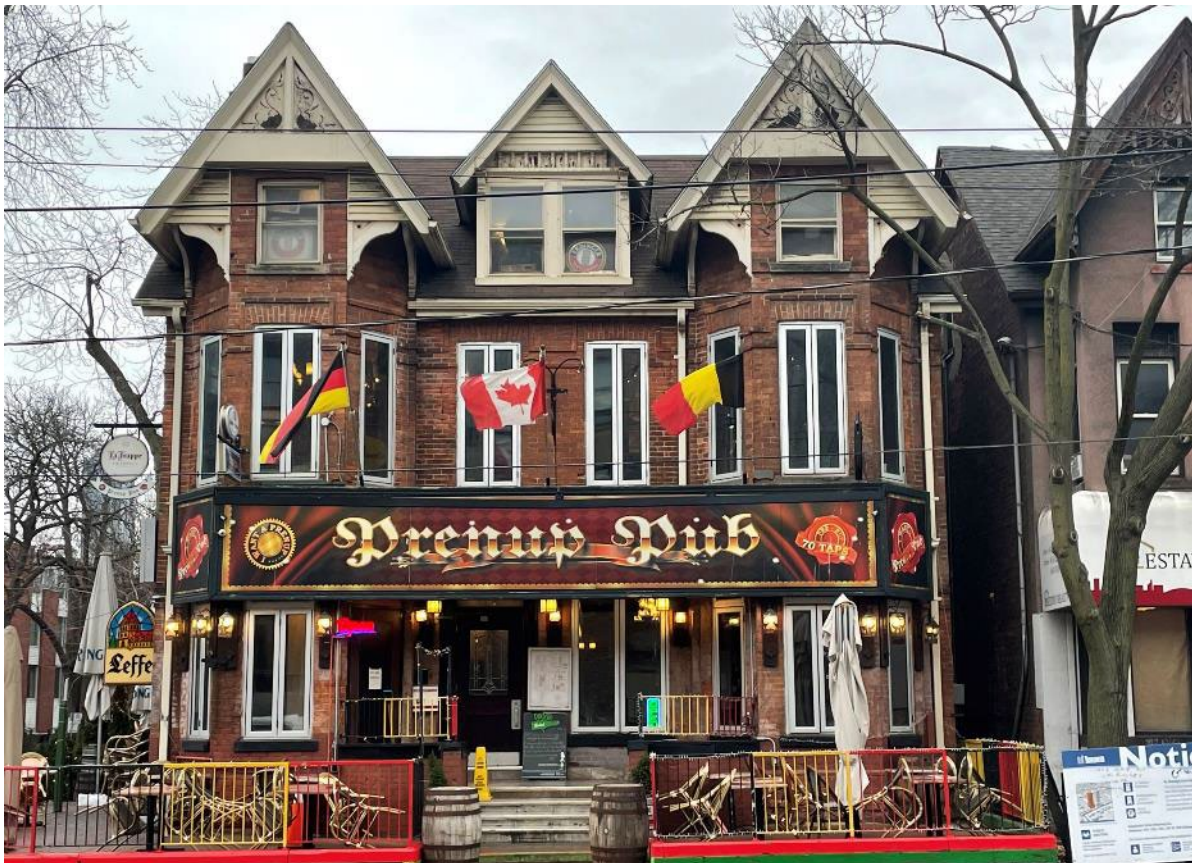
View of North/College Street Elevation of 191 College Street (Heritage Planning, 2022)
