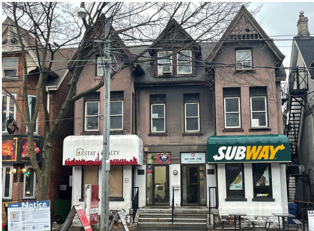
View of North/College Street Elevation of 193-195 College Street (Heritage Planning, 2022)
