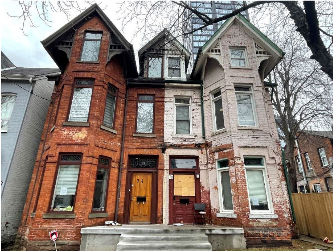
View of Front/East elevation of 74-76 Henry Street (Heritage Planning, 2022)
