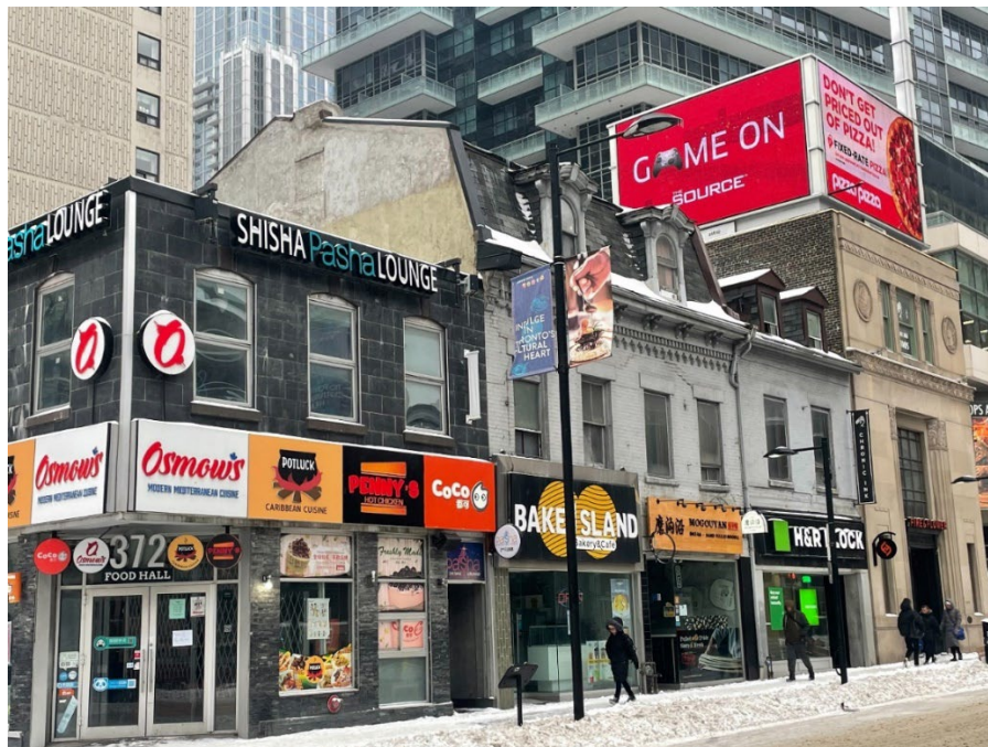
Contextual photograph showing the location of the subject property on the west side of Yonge Street, south of Gerrard Street. Note condition of 372 Yonge Street (left). (Heritage Planning)
