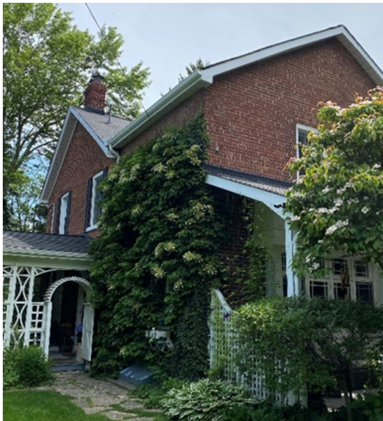
10. View of 24 Mason Blvd. looking southwest, showing the integration of the rear wing (west) with the north elevation (Heritage Planning, 2023).
