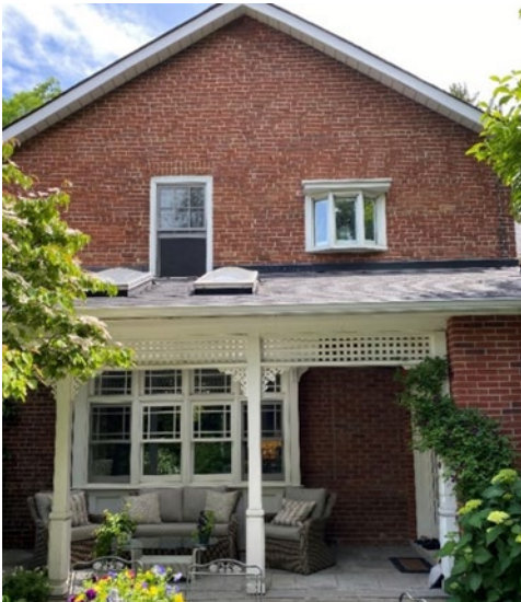
12. Partial view of the west elevation rear wing showing the non-original porch and bay windows. To the lower right is part of the one-storey rear addition with the entrance into the family room (Heritage Planning, 2023).
