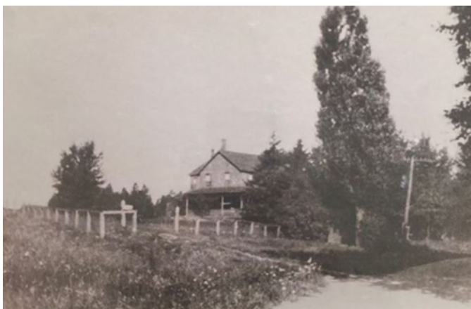
4. Partial view of the south elevation of 24 Mason Blvd. in 1915 showing the original verandah and part of the rear wing addition to the left of the building. Note that the rear wing once had a chimney; this was removed in 1999 (Ted Chirside, North York Historical Society).
