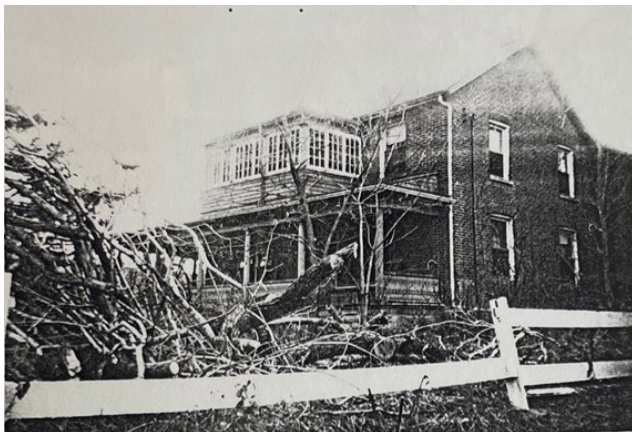
6. View of the east and north elevations of 24 Mason Blvd showing the original verandah, the sleeping porch, and the original configuration of the windows on the north elevation (North York Historical Society, 1966, NYCL).
