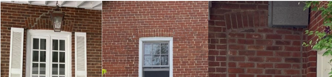
13. Detail comparison of the jack arch brick voussoirs on the original portion of the subject property (at far left) and the varied segmental arch brick voussoirs on the rear wing (Heritage Planning, 2023).
