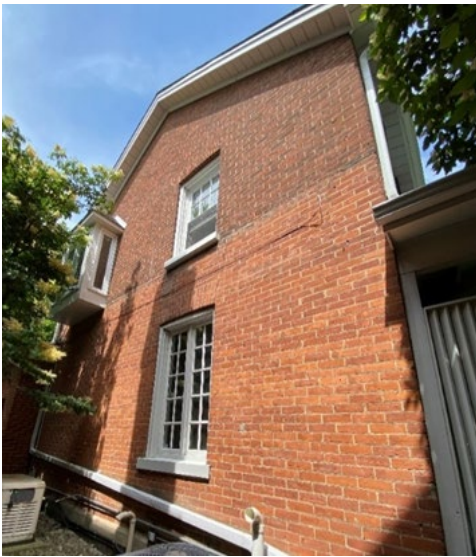
11. Partial view of the south elevation showing the ghost line of the former verandah, the two original flat or jack arch voussoirs, and the non-original bay window. The former south elevation entrance, beneath the bay window, has been bricked over (Heritage Planning, 2023).
