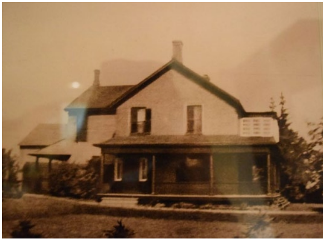
5. Historic photo of 24 Mason Blvd., taken between 1930-1970, showing the south elevation with original verandah and the earliest confirmed entrance at lower left, and the sleeping porch at upper right. The rear (west) wing addition is also visible (Photo provided by property owners, n.d., estimated date range determined by historical aerials and the post-1970 alterations).
