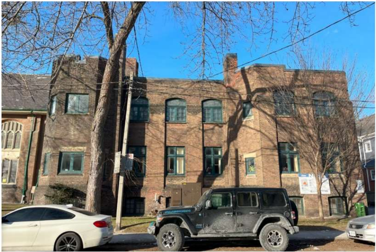
Figure 8. Photograph showing the Sunday School wing of St. John's Presbyterian Church (looking north) at the rear of the property (ERA Architects Inc., 2024).
