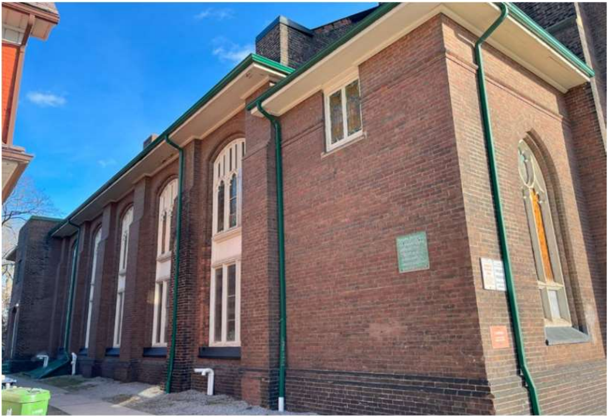
Figure 7. Photograph showing the nave portion of the north elevation of St. John's Presbyterian Church (ERA Architects Inc., 2024).
