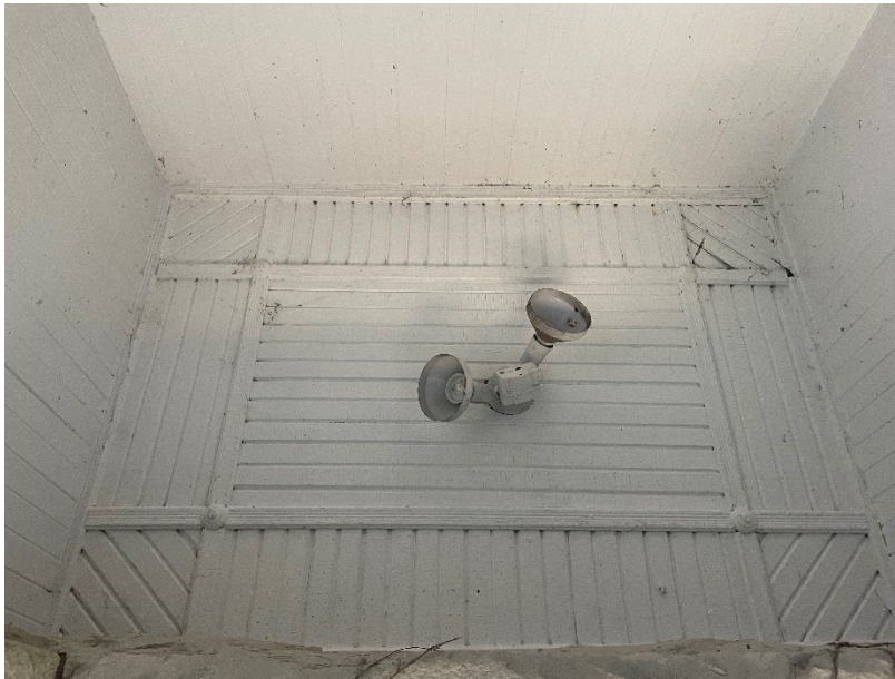
Figure 19: 6 Cawthra Square recessed entry showing Queen Anne-style, wood-paneled tongue-and-groove wall and ceiling cladding. 8 Cawthra Square retains the same entry ceiling detail although the wall panelling has been lost or covered, 2023 (City of Toronto Heritage Planning)
