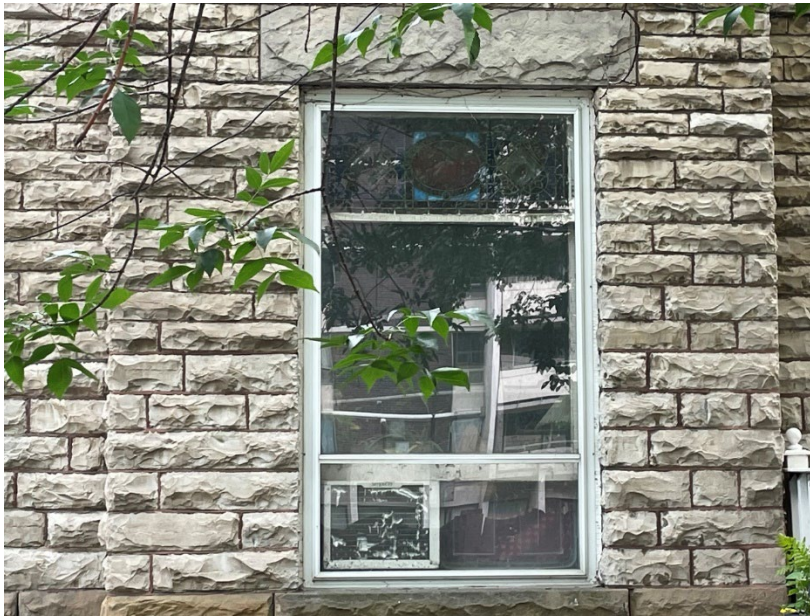
Figure 17: 6 Cawthra Square, detail view showing an example of the window sashes with leaded and stained glass transom light (behind modern storm sash), 2023 (City of Toronto Heritage Planning)
