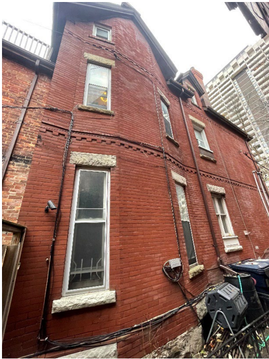
Figure 15: 6 Cawthra Square, portion of east façade, 2023 (City of Toronto Heritage Planning)
