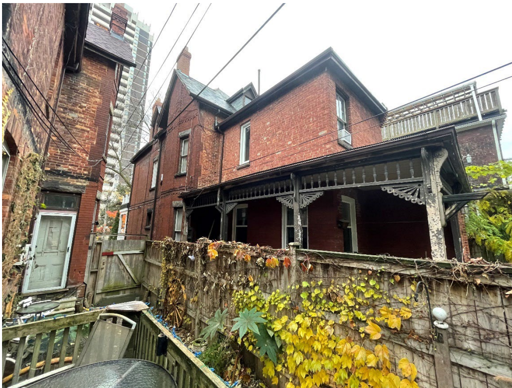
Figure 23: 8 Cawthra Square, east and rear (north) façades showing rear verandah with spindle work detailing, 2023 (City of Toronto Heritage Planning)
