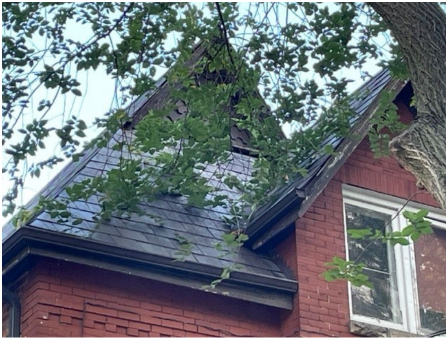
Figure 28: 8 Cawthra Square roofline showing front gable and gable-on-hip roof and shingle cladding within gable (inverse roofline of 6 Cawthra Square), 2023 (City of Toronto Heritage Planning)
