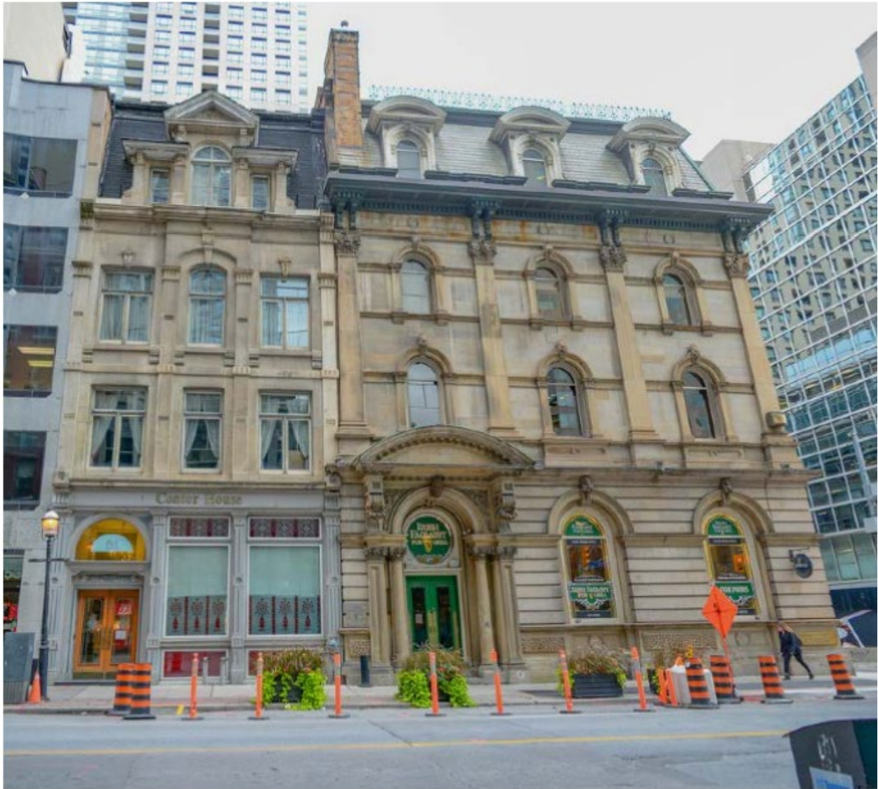
Principal (West) Elevation of 49-51 Yonge Street (Source: HIA prepared by GBCA Architects Ltd., 2021).
