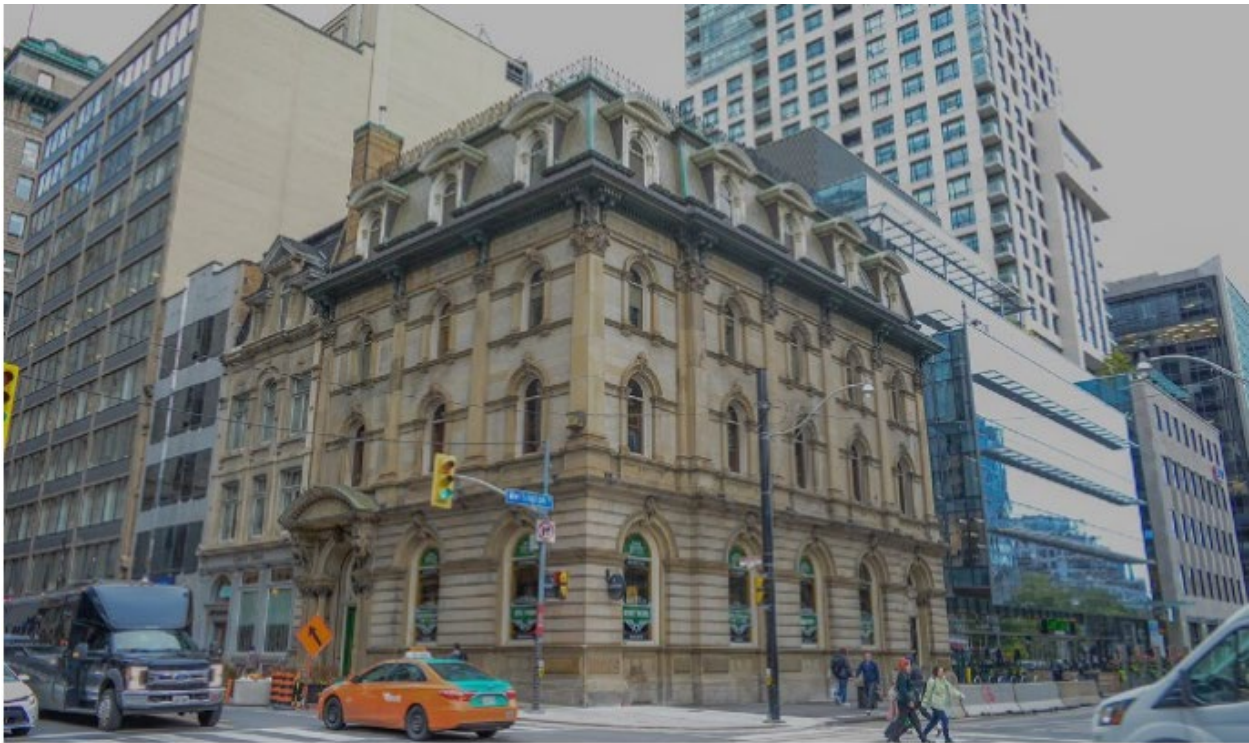
Principal (West) and South Elevations of 49-51 Yonge Street (Source: HIA prepared by GBCA Architects Ltd., 2021).
