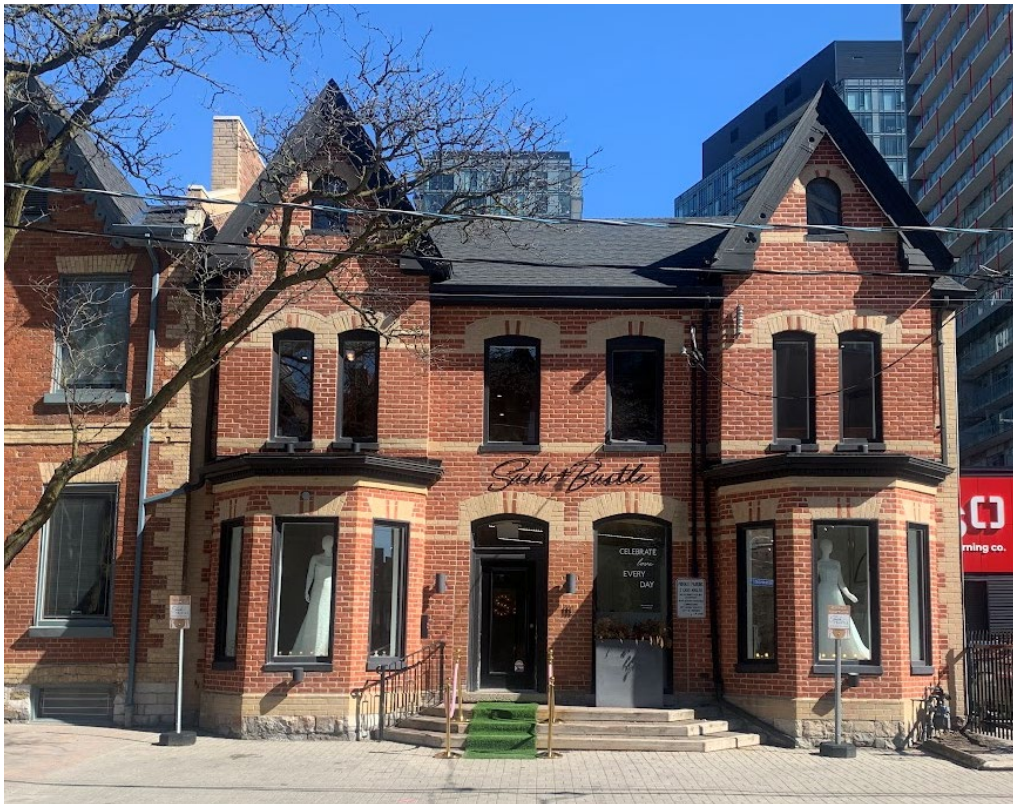
Figure 4. West elevation of 111 Berkeley Street (Heritage Planning, 2024)
