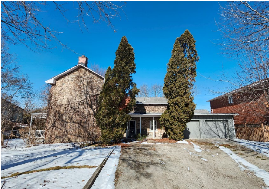
Figure 15. Detail of the current primary (south) elevation fronting La Rose Avenue with the main entrance in the centre and the modern 2-bay garage on the right (Heritage Planning, 2024)
