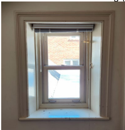
Figure 28. Detail of the casement of the window in the second storey of the side (east) wall of the rear kitchen wing (Heritage Planning, 2024)
