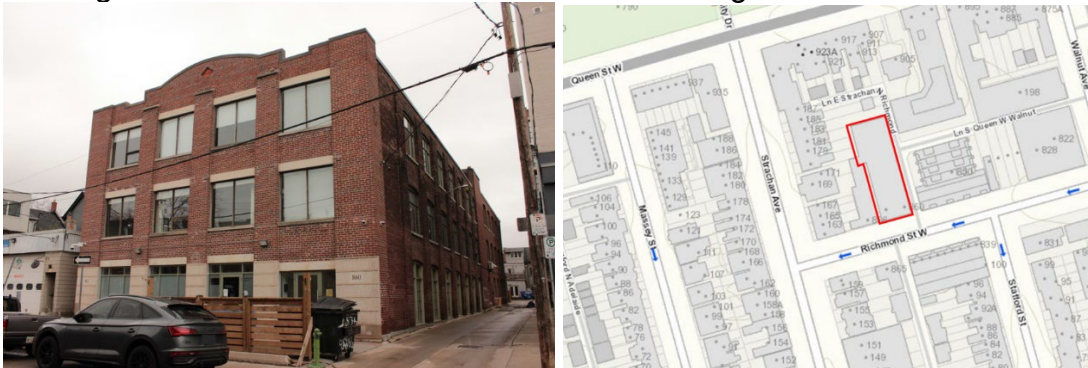
860 Richmond Street West (Heritage Planning, 2024). 860 Richmond Street West (indicated in red).
