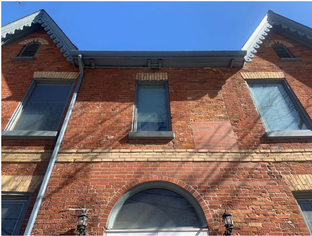
Figure 10. Detail of west elevation at 115 Berkeley Street showing an infilled opening at the second storey and differentiation of brickwork around the main entrance (Heritage Planning, 2024)
