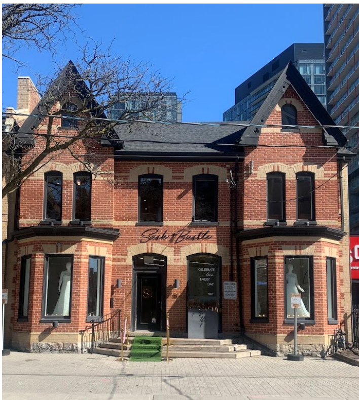
111 Berkeley Street (Heritage Planning, 2024)
