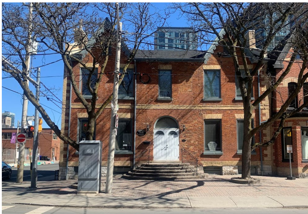
Figure 9. West elevation of 115 Berkeley Street (Heritage Planning, 2024)
