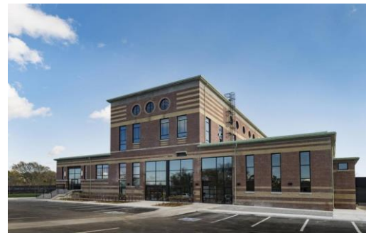
Symes Road Incinerator (Image source: 5iv15fteen via ACO TO Built)
